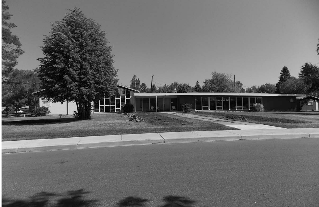
Looking north at the site from 109A Avenue and 139 Street
