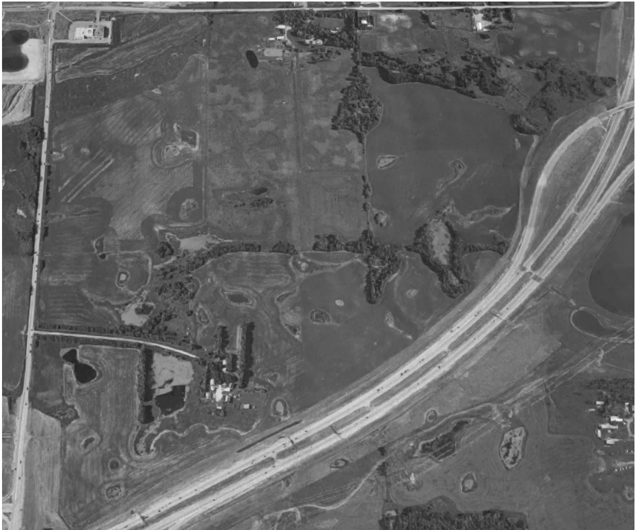
Figure 2: the south area of the proposed Aster NSP, with the present 23 Avenue NW along the top, the existing church in the upper left, and Anthony Henday Drive running along the right and bottom
