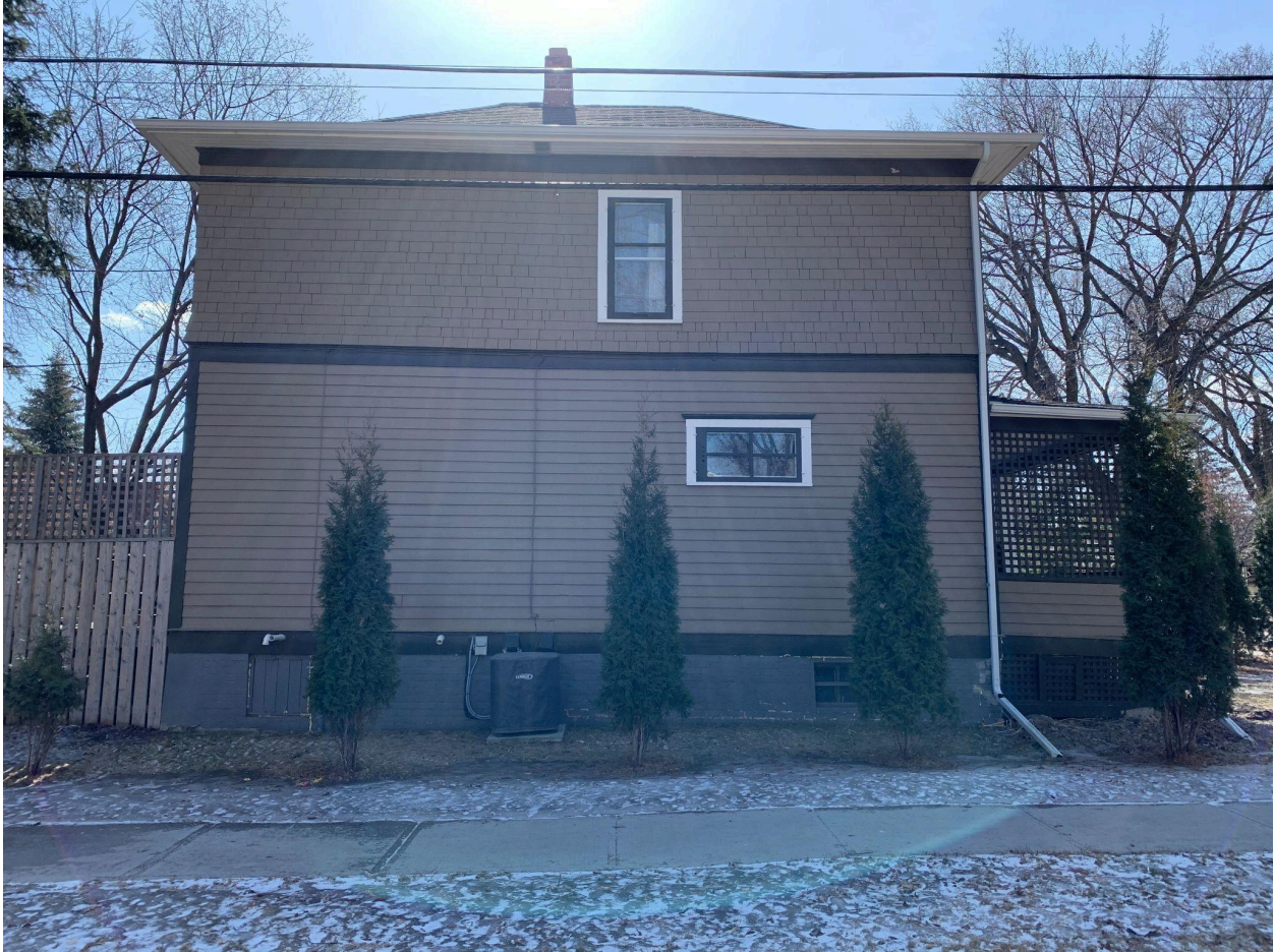
View of north elevation, looking south from 106 Avenue NW.
