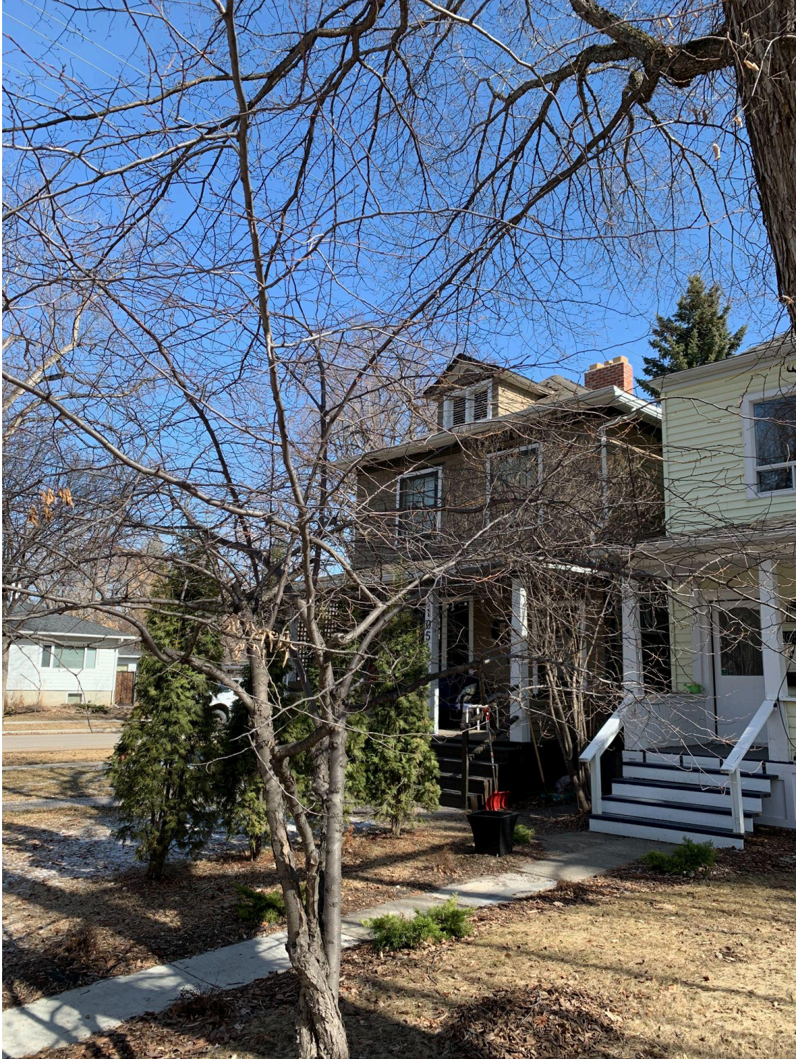
View of south and west elevations, looking northeast from 126 Street NW.
