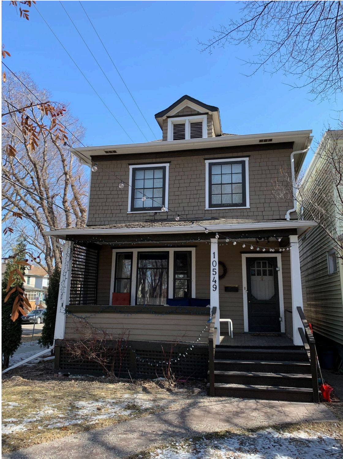
View of west elevation, looking east from 126 Street NW.
