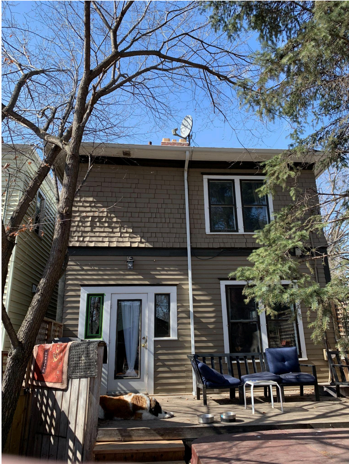
View of east elevation, looking west from property rear yard.
