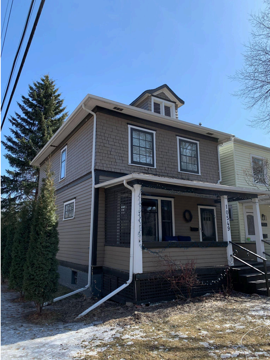
View of west (front) and north (side) elevations, looking southeast from 126 Street NW.
