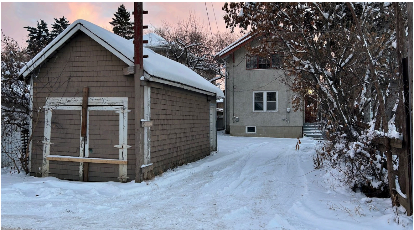
View of site looking south from alley
