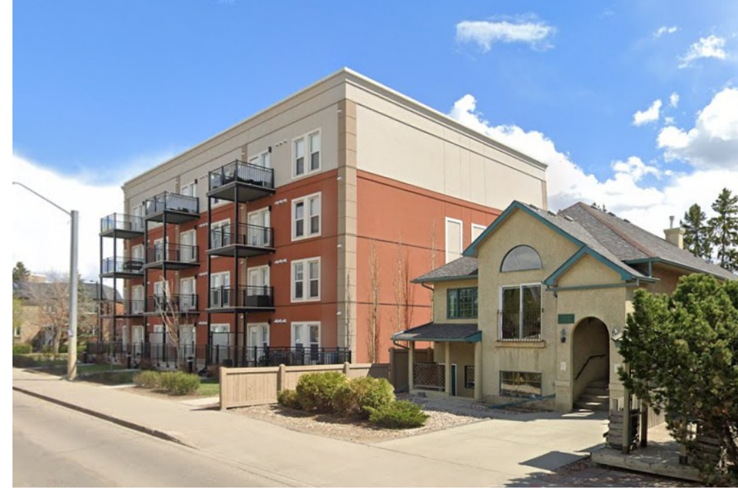
4-Storey Precedent Building – 14411 Stony Plain Road
