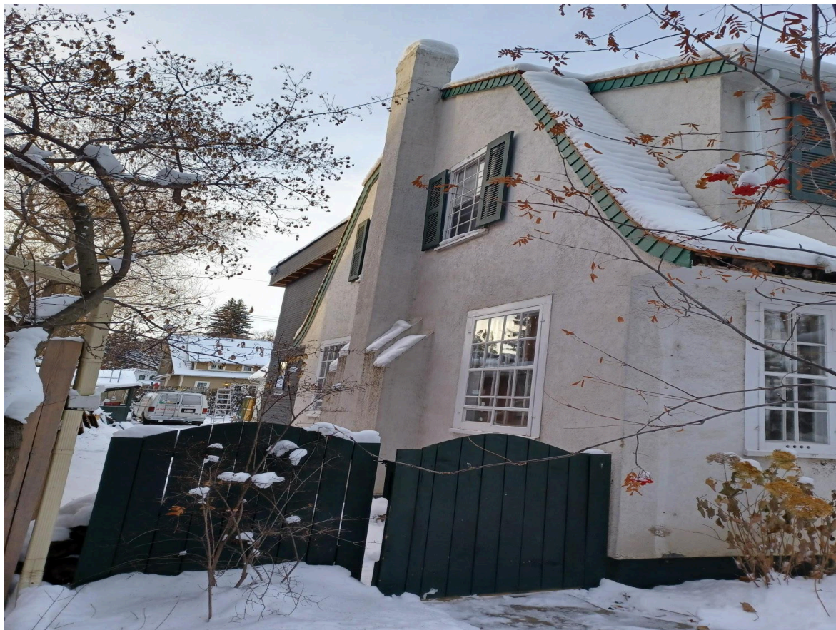
View of side (south) elevation, looking northwest from property front yard. Note new addition at the rear of the building (the rear elevation is not included in the designation).
