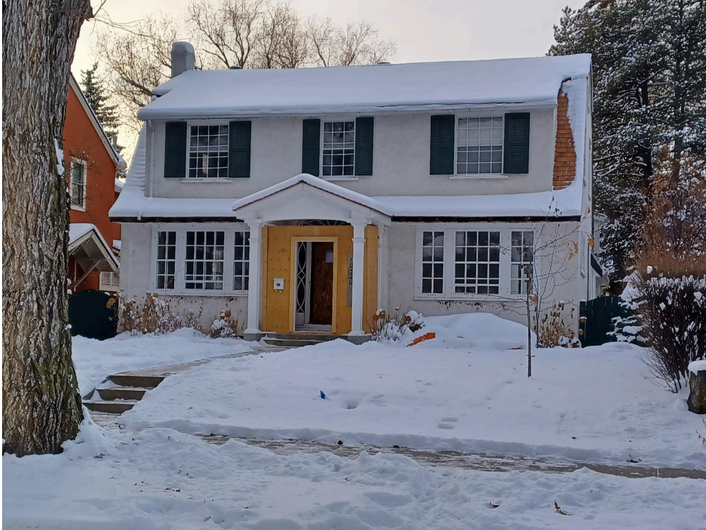
View of front (east) elevation, looking west from 132 Street NW.
