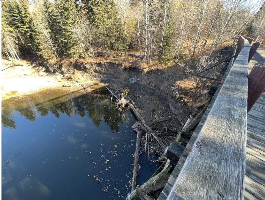
Photo 27: View downstream from trestle bridge, showing significant bank instability (October 20, 2022, UTM 336237E/593211N).
