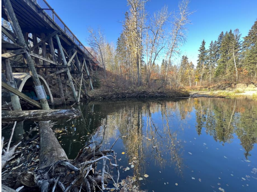
Photo 32: View of scour pool below culvert (October 20, 2022, UTM 336249E/5932126N).
