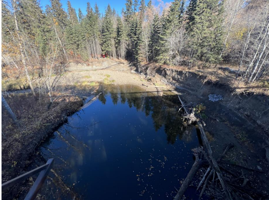
Photo 26: View downstream from trestle bridge, showing large scour pool downstream of culvert (October 20, 2022, UTM 336237E/5932111N).
