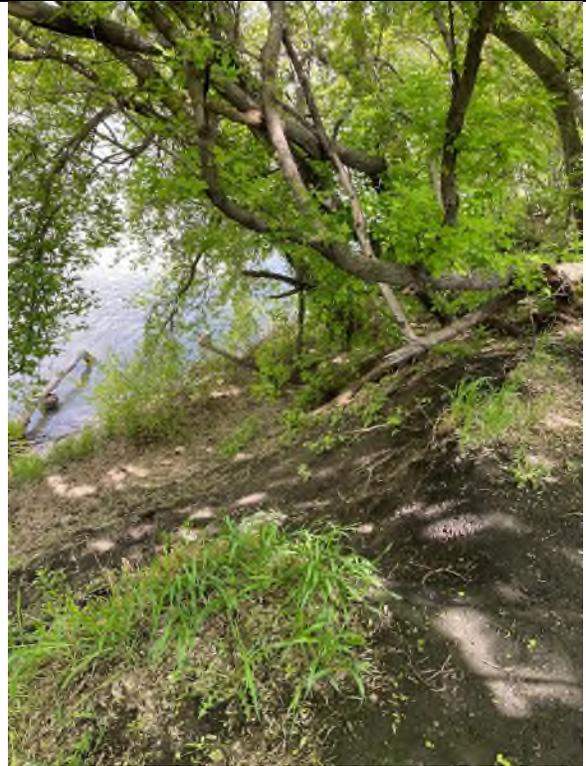
Picture 14: toe of slope, leaning trees/bare soil
