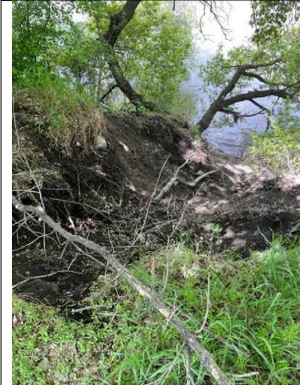
Picture 13: erosion at toe of slope along river
