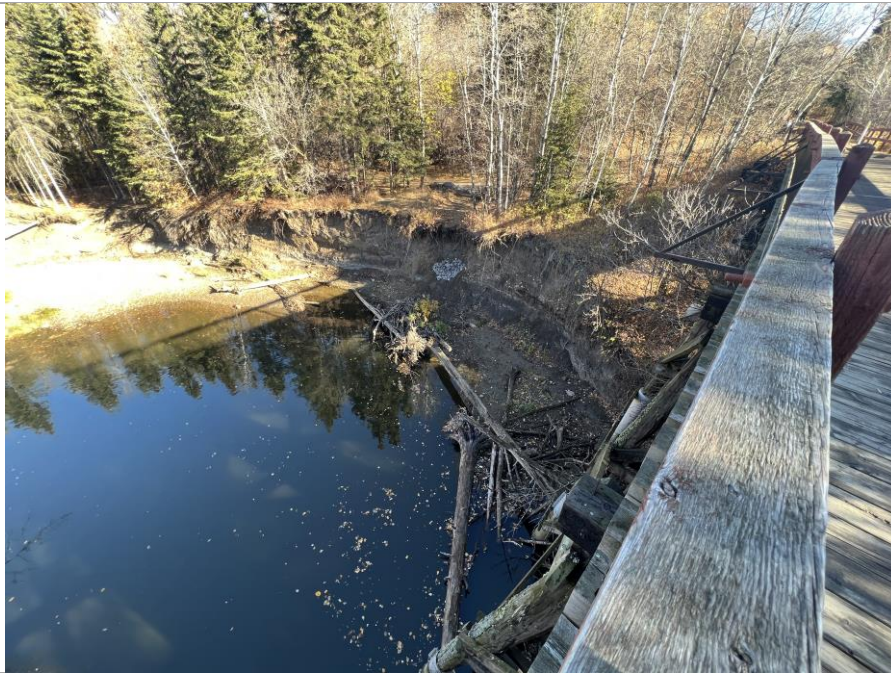
Photo 27: View downstream from trestle bridge, showing significant bank instability (October 20, 2022, UTM 336237E/5932111N).
