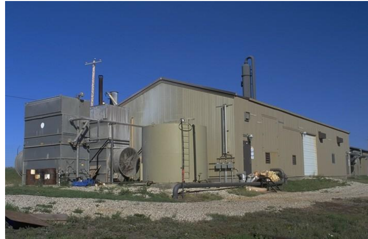
Landfill Gas Collection Facility
