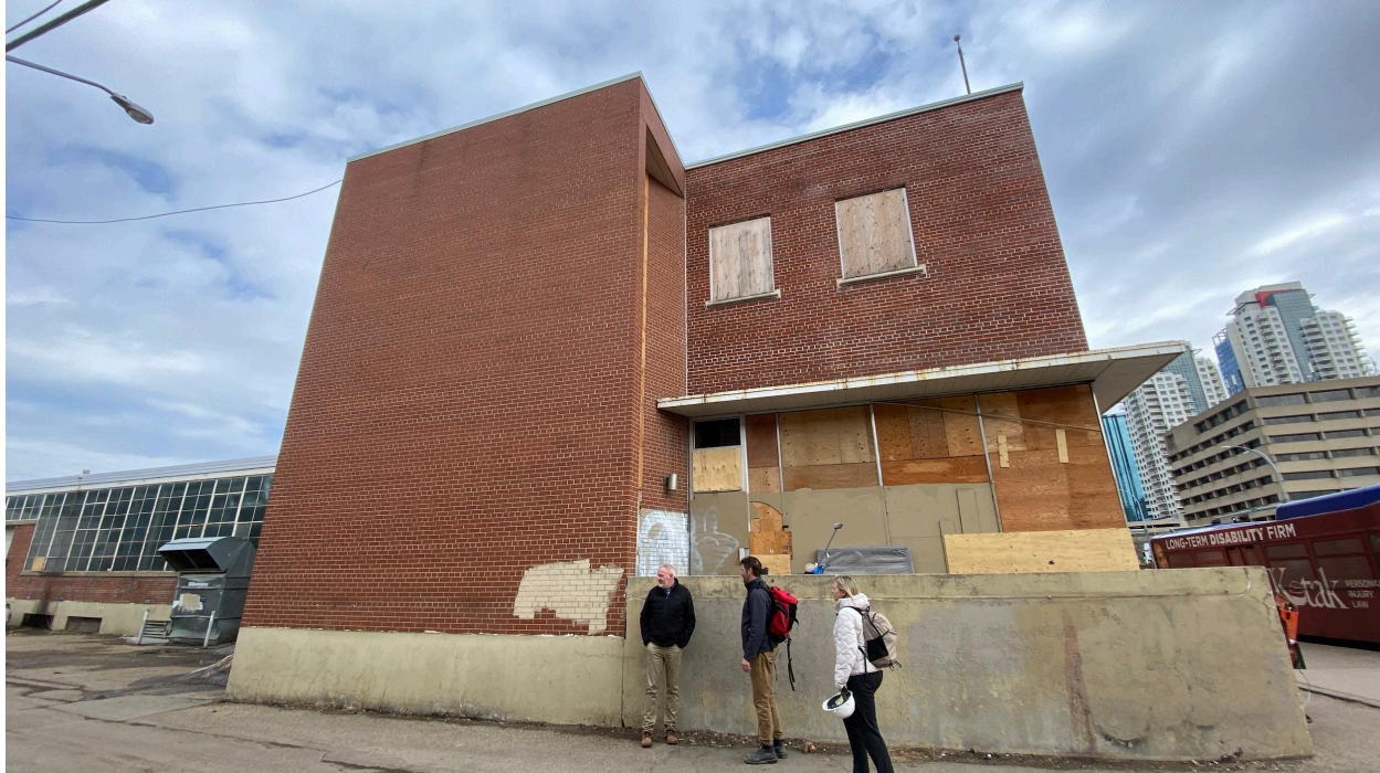
View of side (west) elevation, looking east from adjacent lane. The lower height addition to the left of the two-storey 1947 building is not part of the designation and will be demolished.
