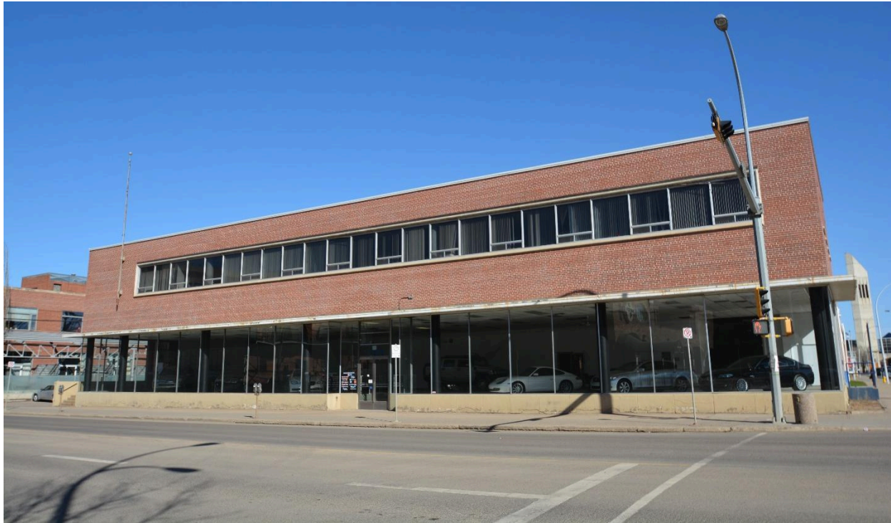
View of front (south elevation), looking north from 103 Avenue NW, in 2015.
