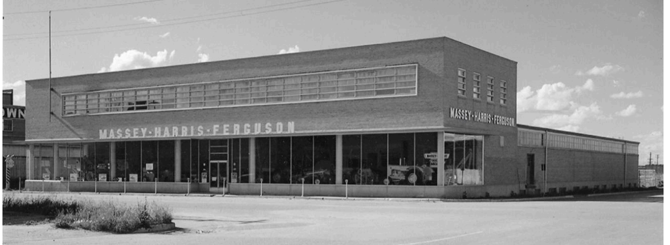
Massey Ferguson Building (then known as the Massey Harris Ferguson Building) in 1953.
