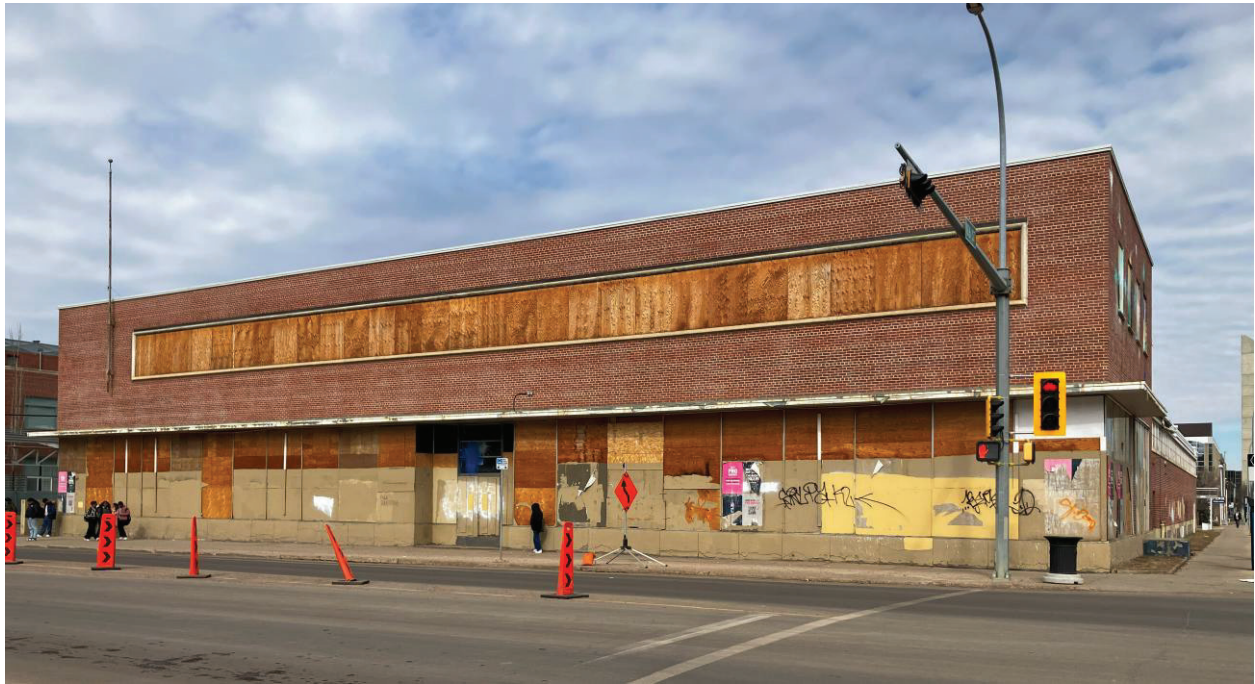
View of front (south) elevation, looking north from 103 Avenue NW.
