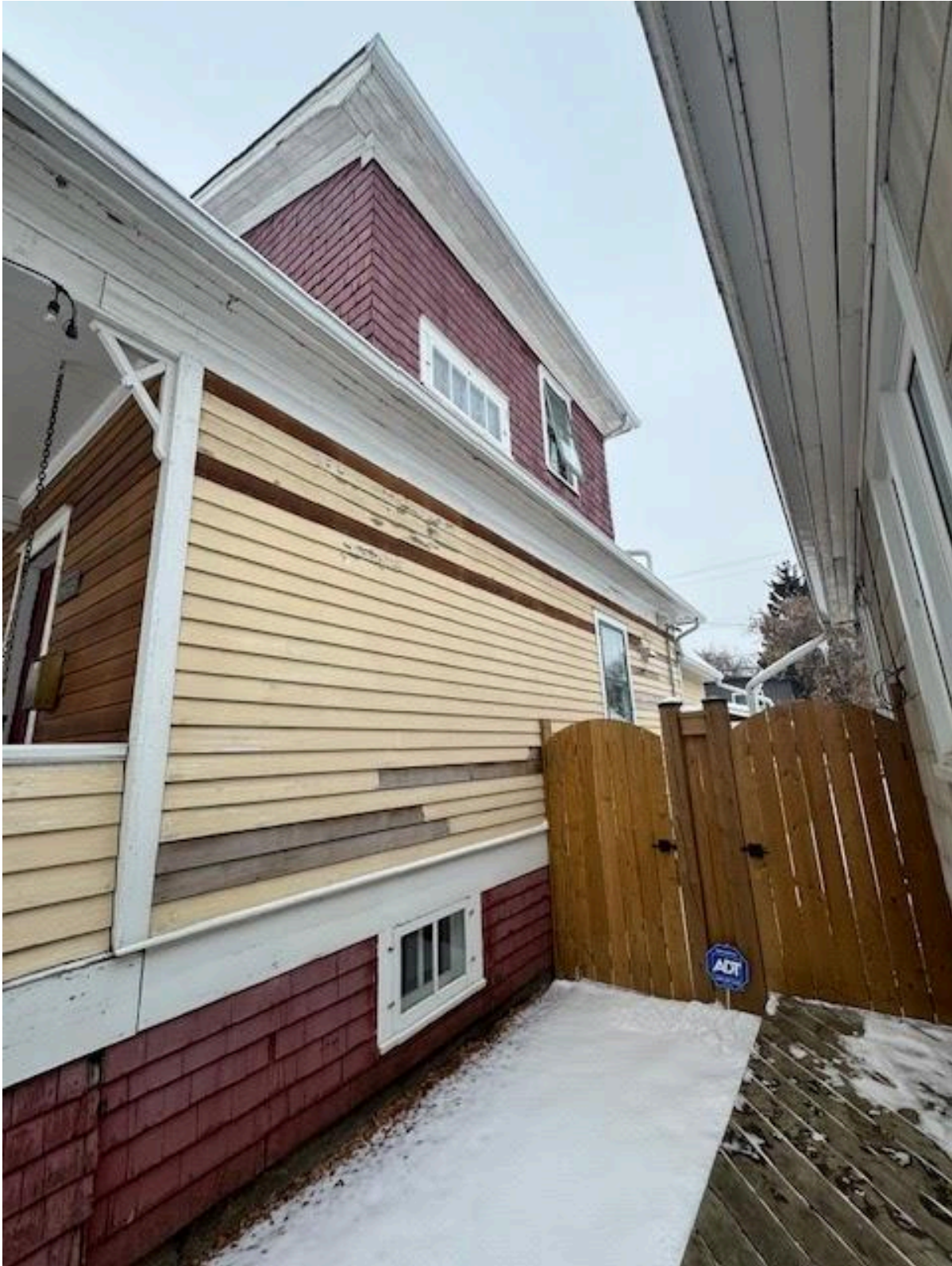
View of side (north) elevation, looking west from the front yard of the property.
