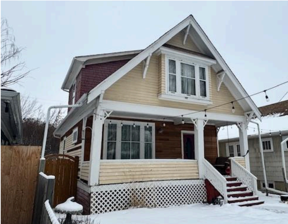
View of front (east) elevation and side (south) elevation, looking northwest from 95a Street NW.
