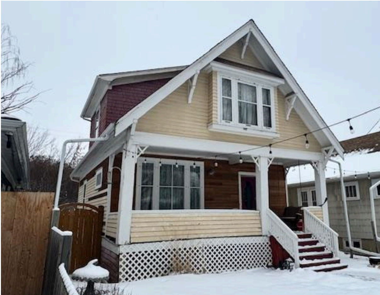
View of front (east) elevation and side (south) elevation, looking northwest from 95a Street NW.
