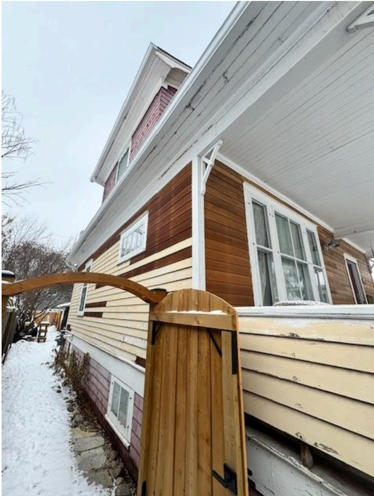
View of side (south) elevation, looking west from the front yard of the property.
