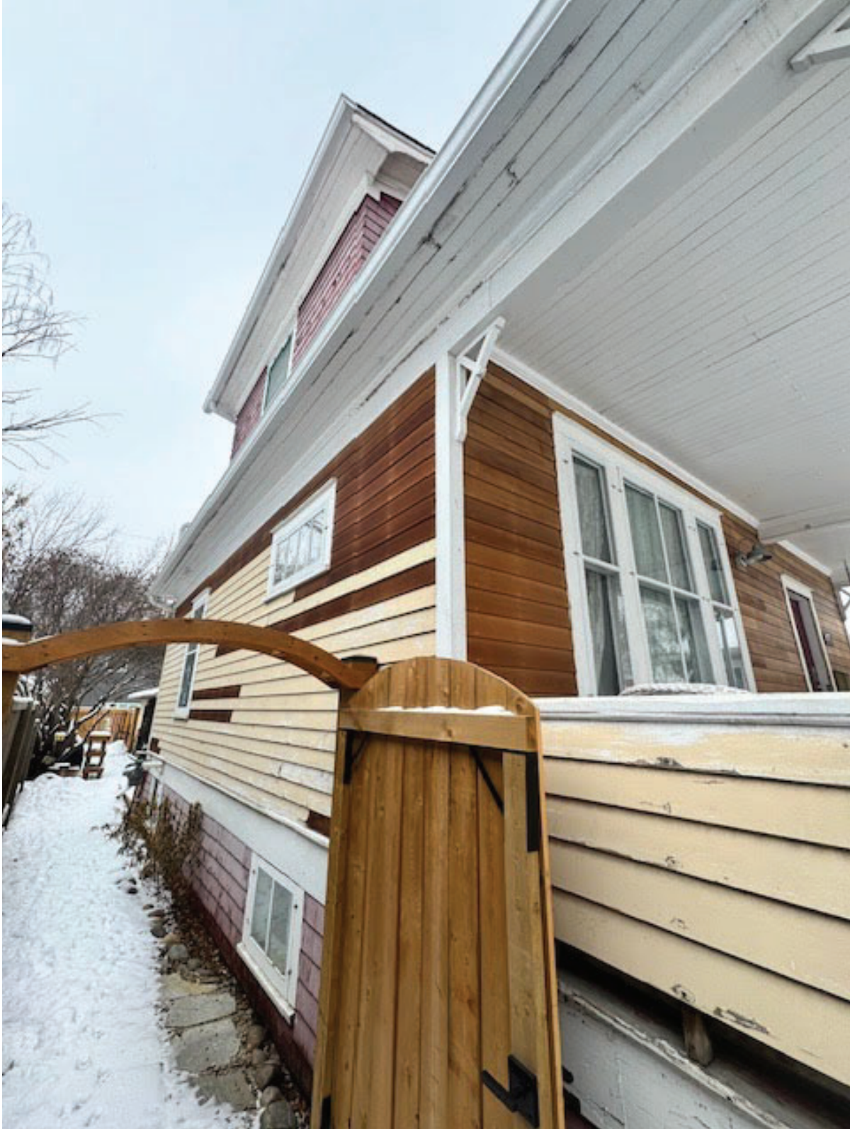
View of side (south) elevation, looking west from the front yard of the property.
