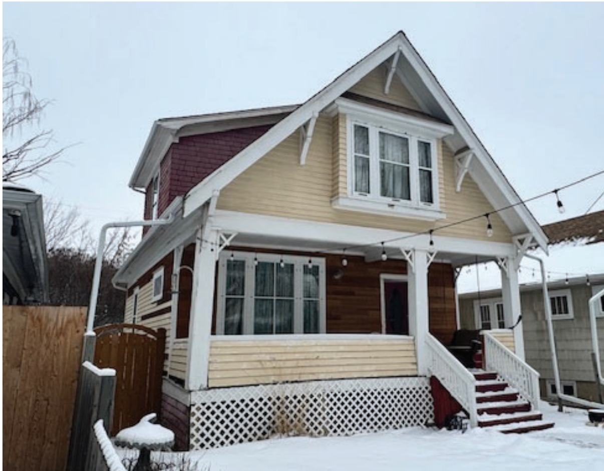
View of front (east) elevation, looking northwest from 95A Street NW.
