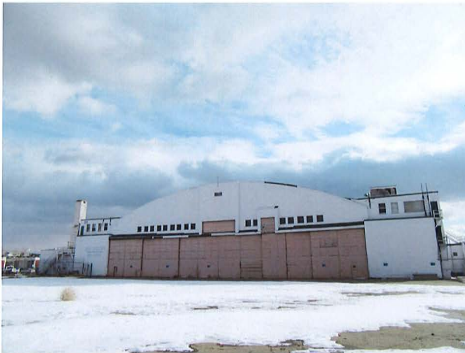
Hangar 11, north elevation, looking southeast from Blatchford site.
