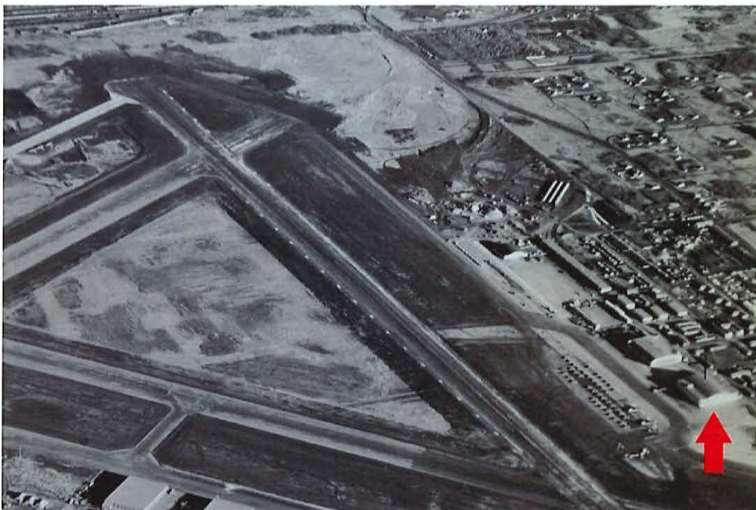
Hangar 11, shown with red arrow, 1943, looking northeast.
