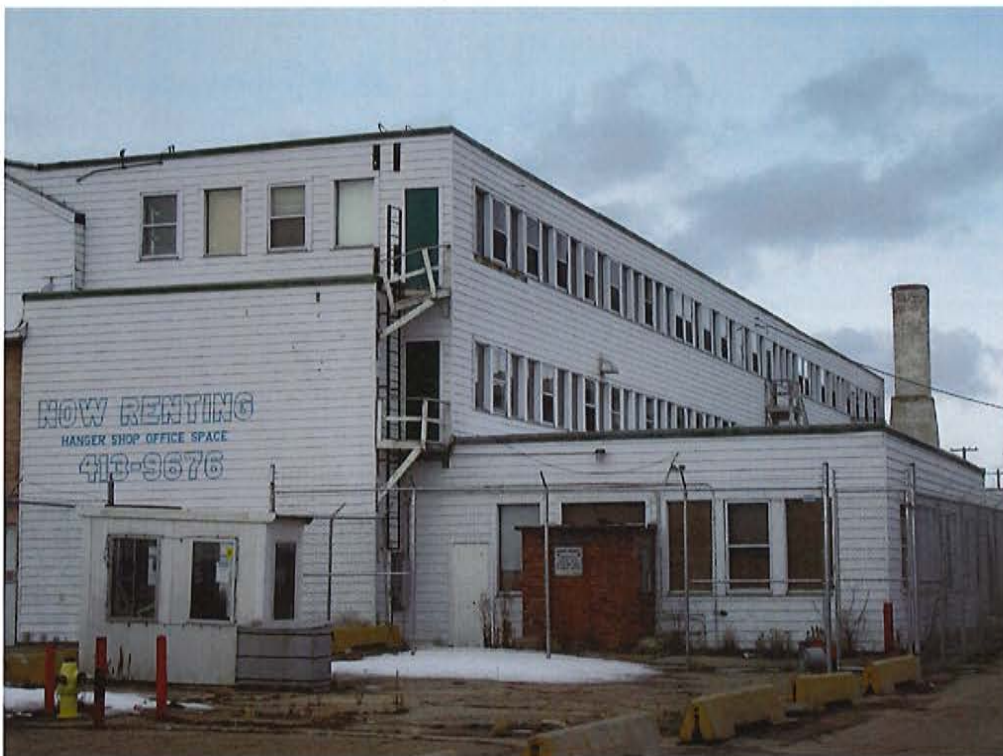
Detail of office wing on east elevation, looking northwest from 109 Street.
