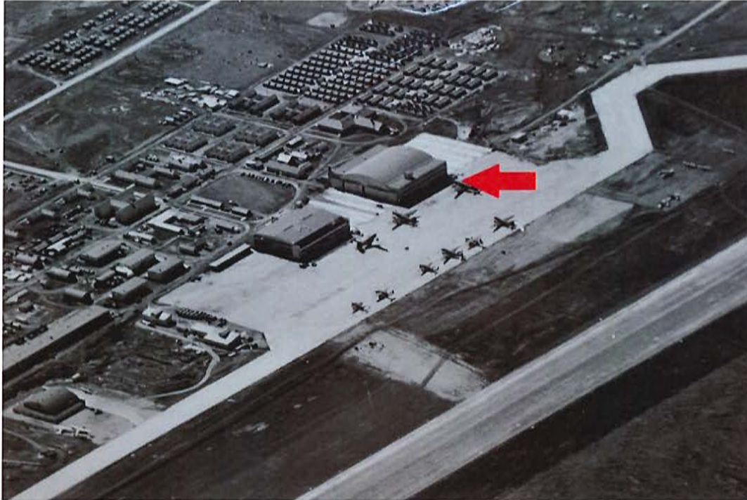
Hangar 11, shown with red arrow, 1943, looking southeast.
