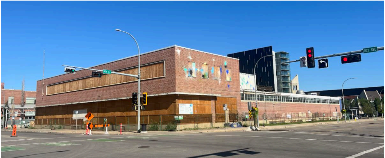
View of the site looking northwest from the intersection of 103 Avenue and 106 Street (Massey Fergus showroom in the foreground)
