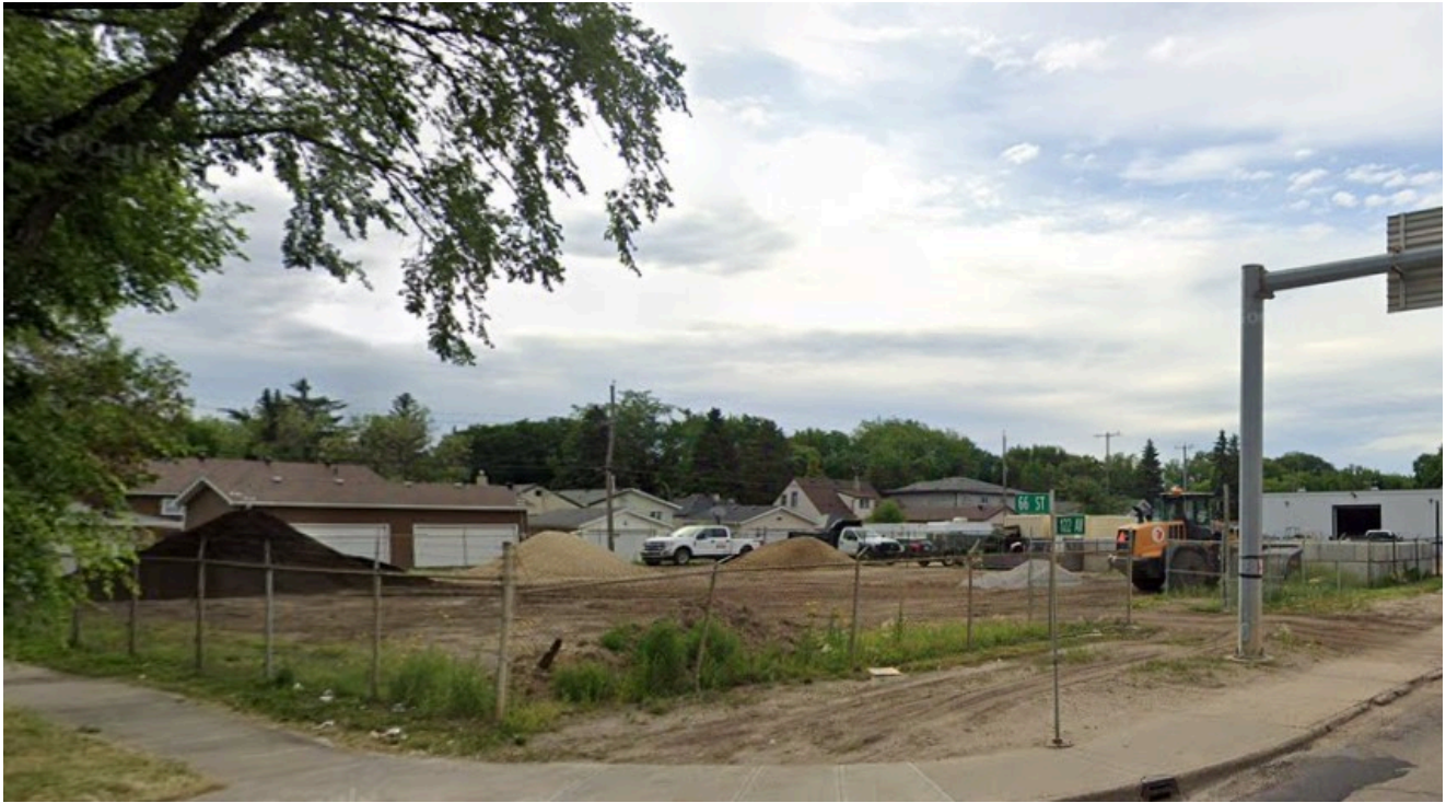
View of the site looking southeast from 66 Street NW & 122 Avenue NW
