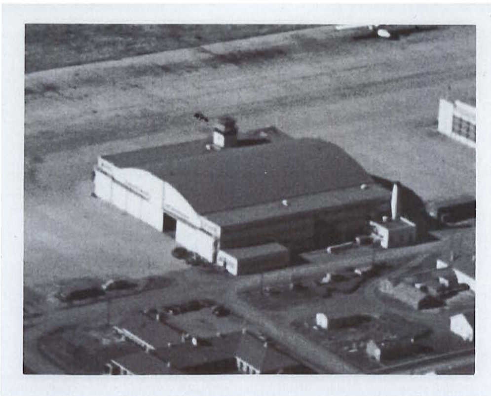
Hangar 11, 1943, looking northwest.
