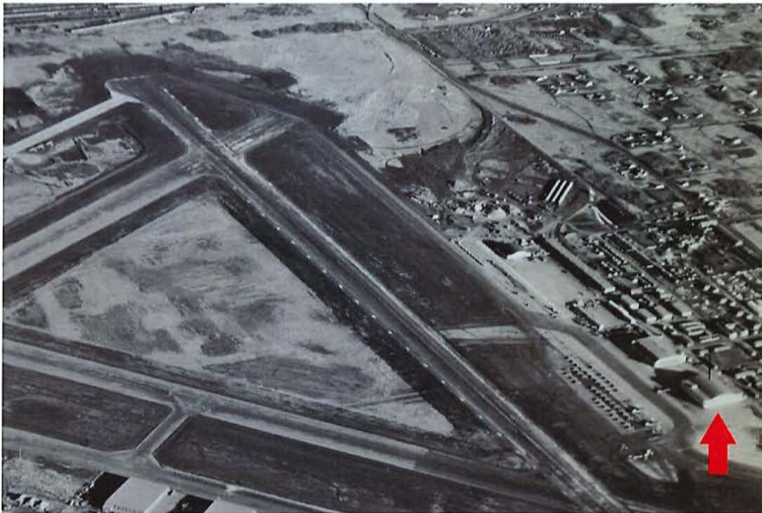
Hangar 11, shown with red arrow, 1943, looking northeast.
