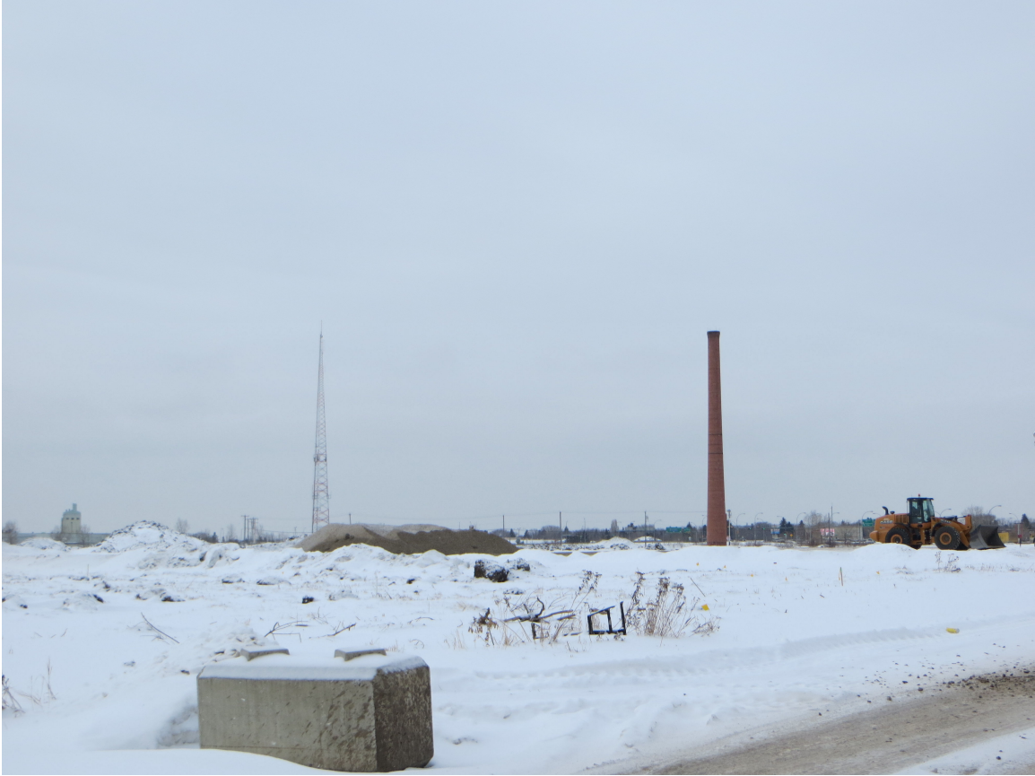
2014, Southeast Elevation (View from 66 Street)
