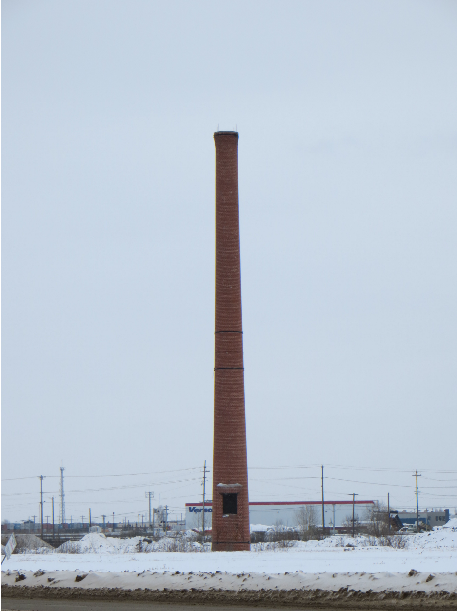
2014, North Elevation (View from Fort Road)
