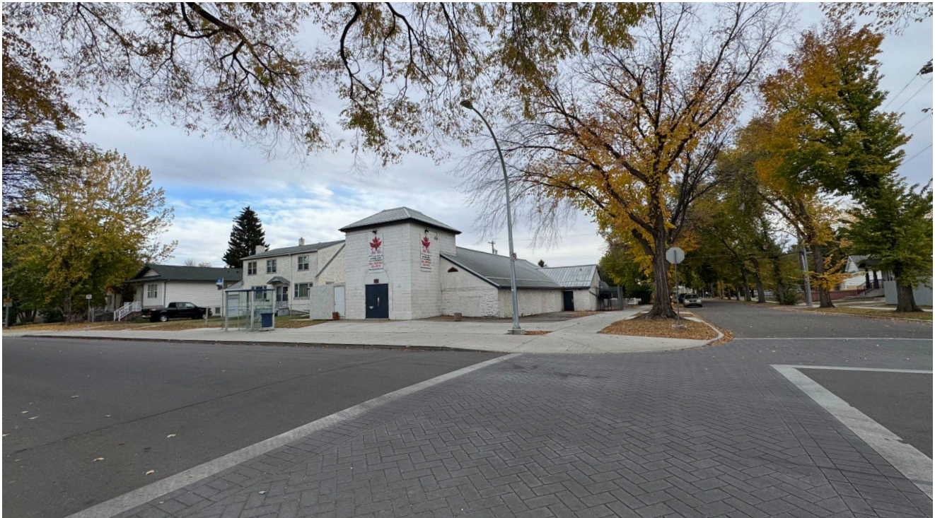
View of site looking south across 129 Ave NW.
