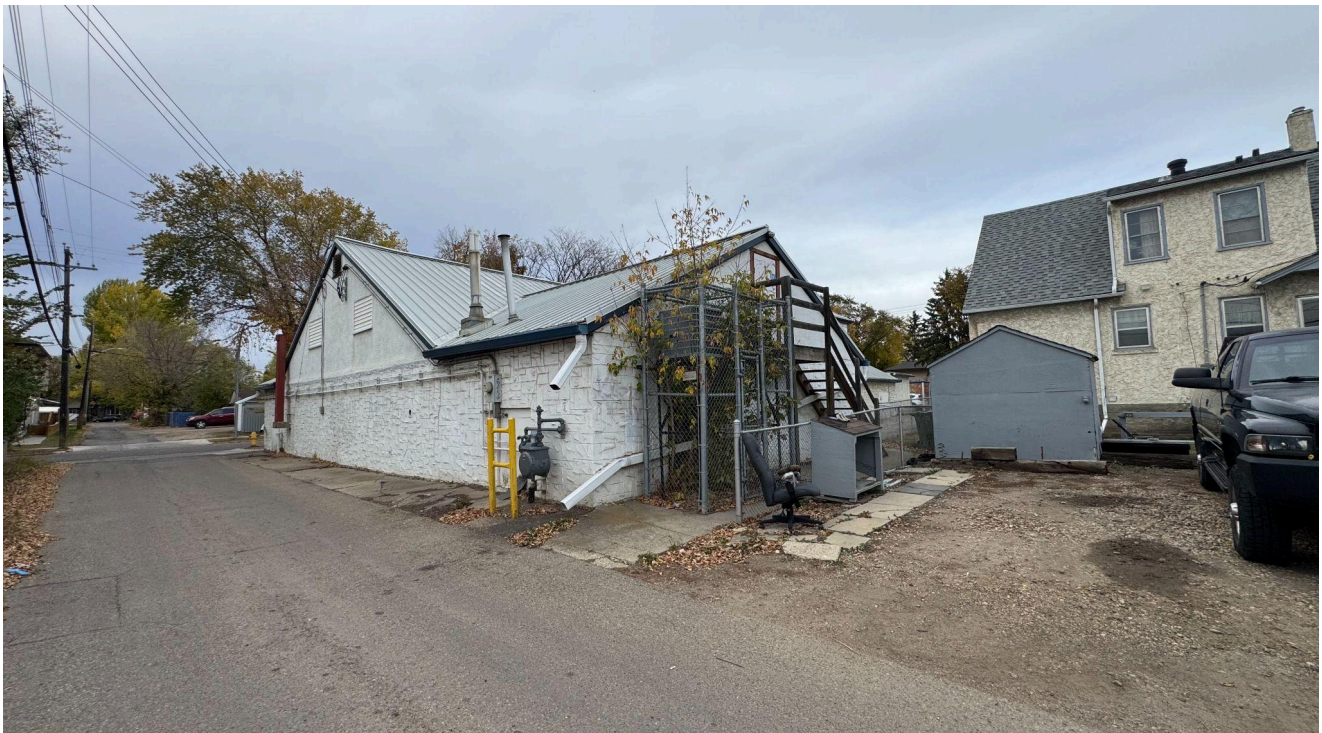
View of site from the rear alley, looking northwest.
