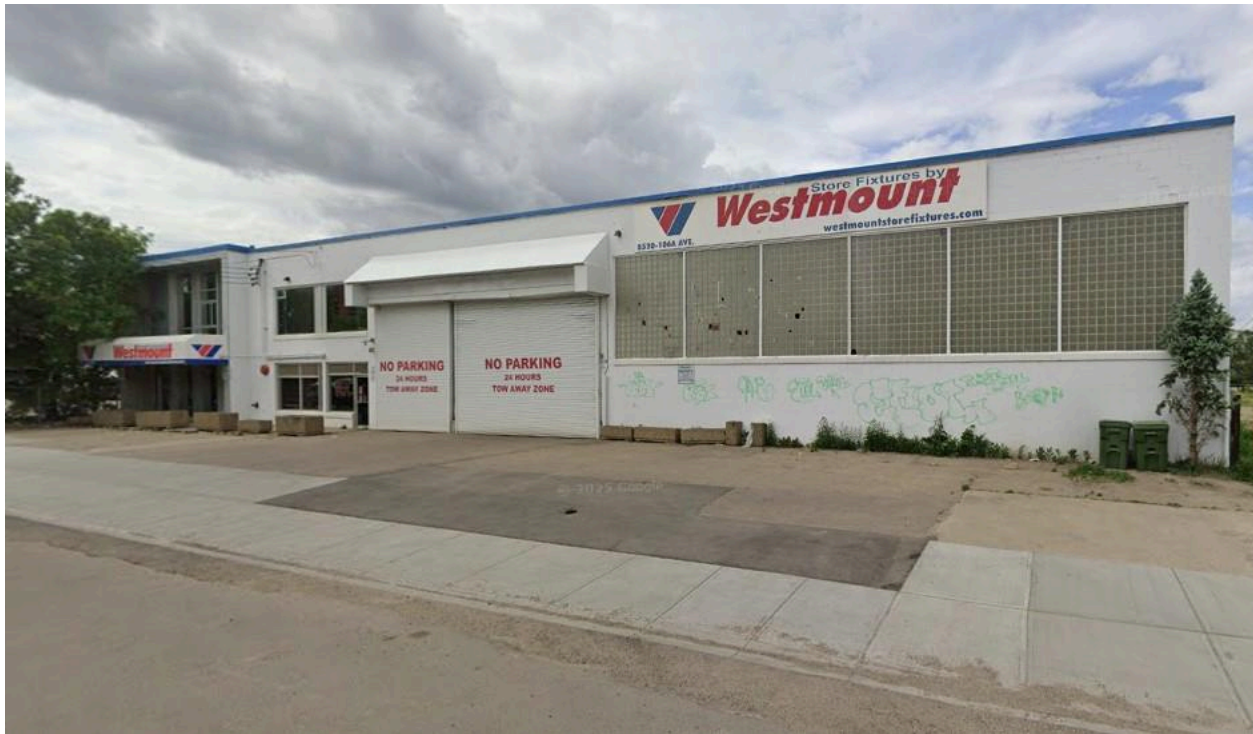
View of the site looking northwest from 106A Avenue NW (Source: Google Maps)
