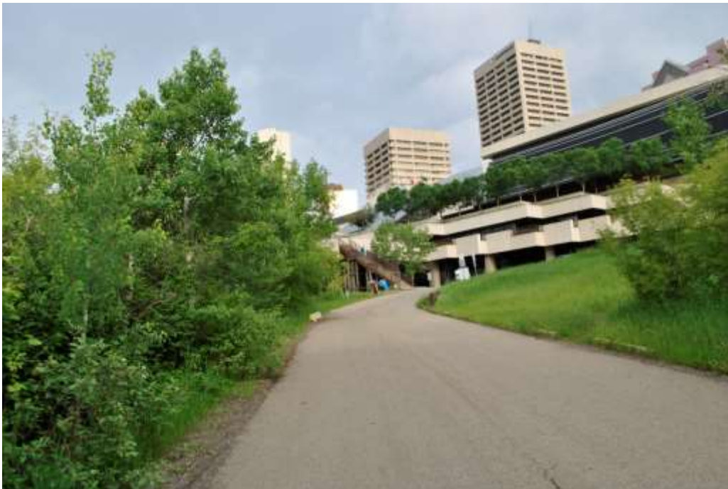
Plate 2.1. Segment of proposed Louise McKinney Riverfront Park Construction Access Road using existing maintenance road, looking northeast.
