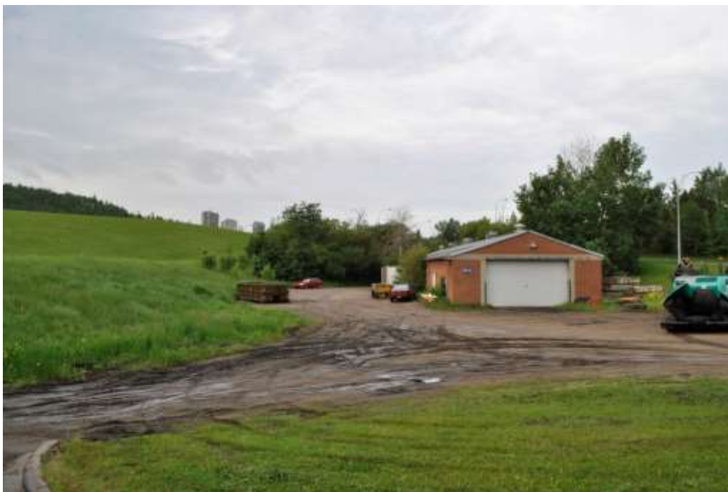
Plate 10.4. Alternative view of existing storage building and surrounding grounds (July 2014).
