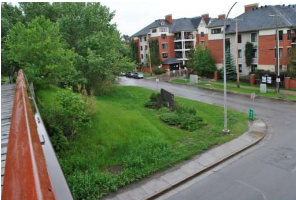
Plate 2.5. Area of proposed boundary changes at HMEP entrance (98 Ave and 96A St), looking northeast (June 2014).
