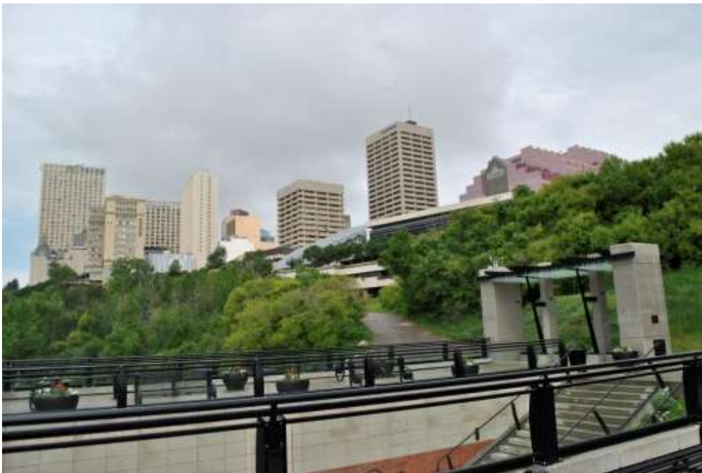
Plate 4.13. West End of proposed primary construction access road, looking northeast towards the maintenance vehicle access road and the Shaw Conference Centre, from the Riverfront Plaza (June 2014).
