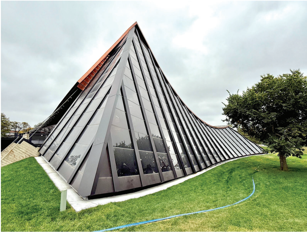
View of west (at right) and north (at left) elevations, looking southeast.
