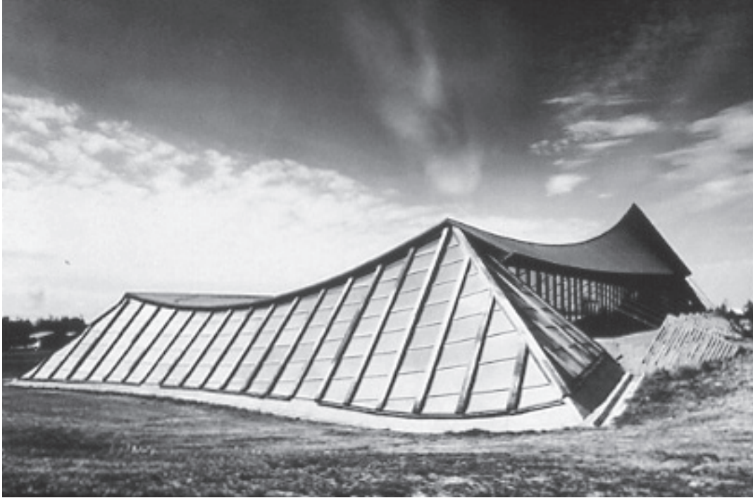
View of east elevation, shortly after completion, circa 1970.
