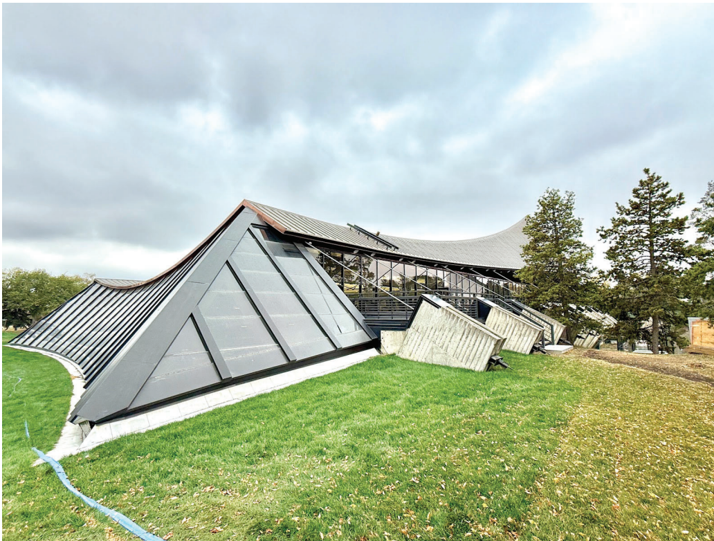
View of north elevation, looking southwest.
