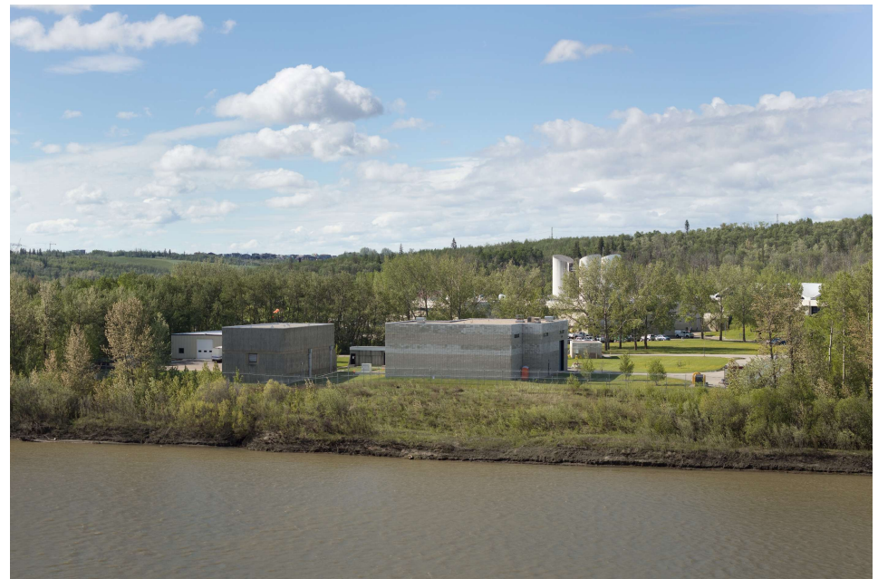
E.L. Smith Water Treatment Plant
