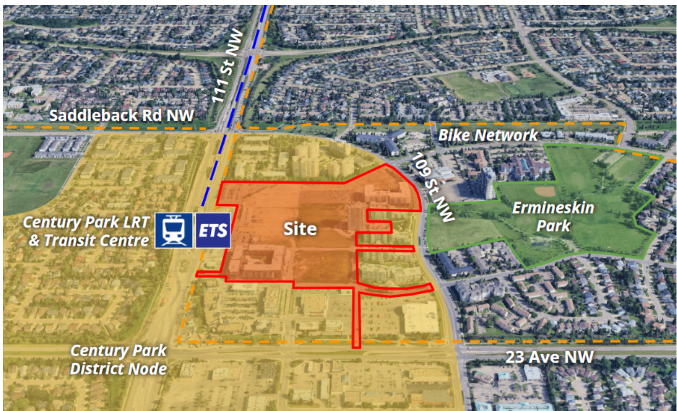
The proposed rezoning site and Special Area boundary with surrounding neighbourhood context
