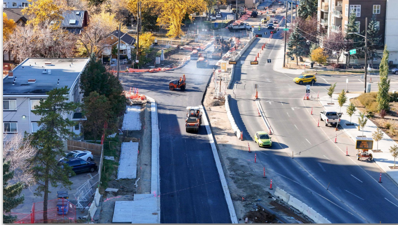
Paving along 104 Avenue
