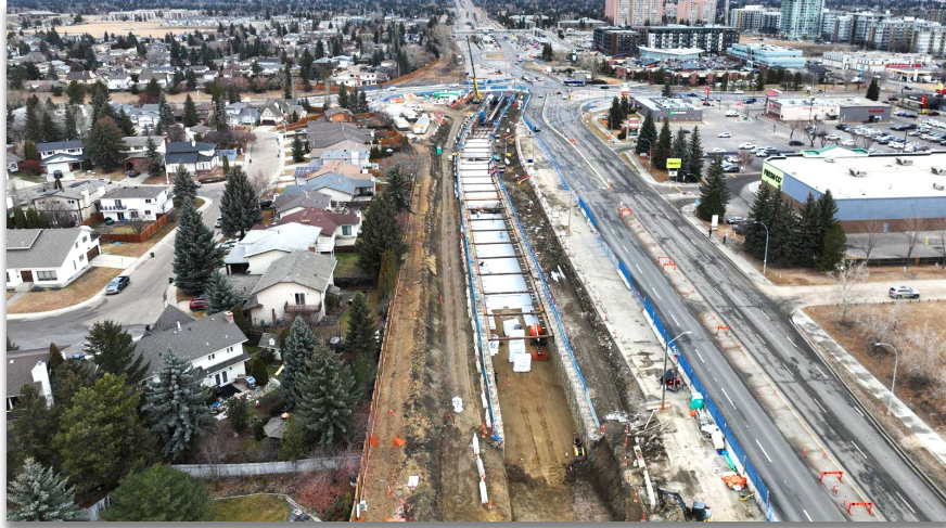
LRT underpass at 23 Ave/111 Street (looking north)
