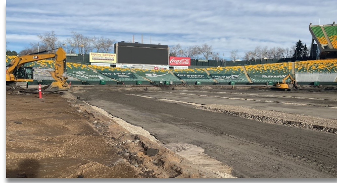
Stadium (Under Construction)
