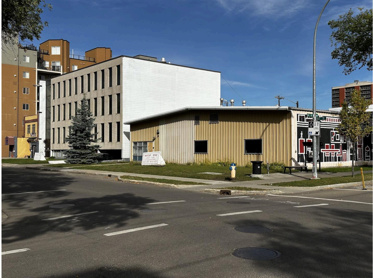
View of front (west) and side (south) elevations, looking northeast from the intersection of 102 Avenue NW and 112 Street NW. The one-storey annex building in the foreground is not part of the designation.
