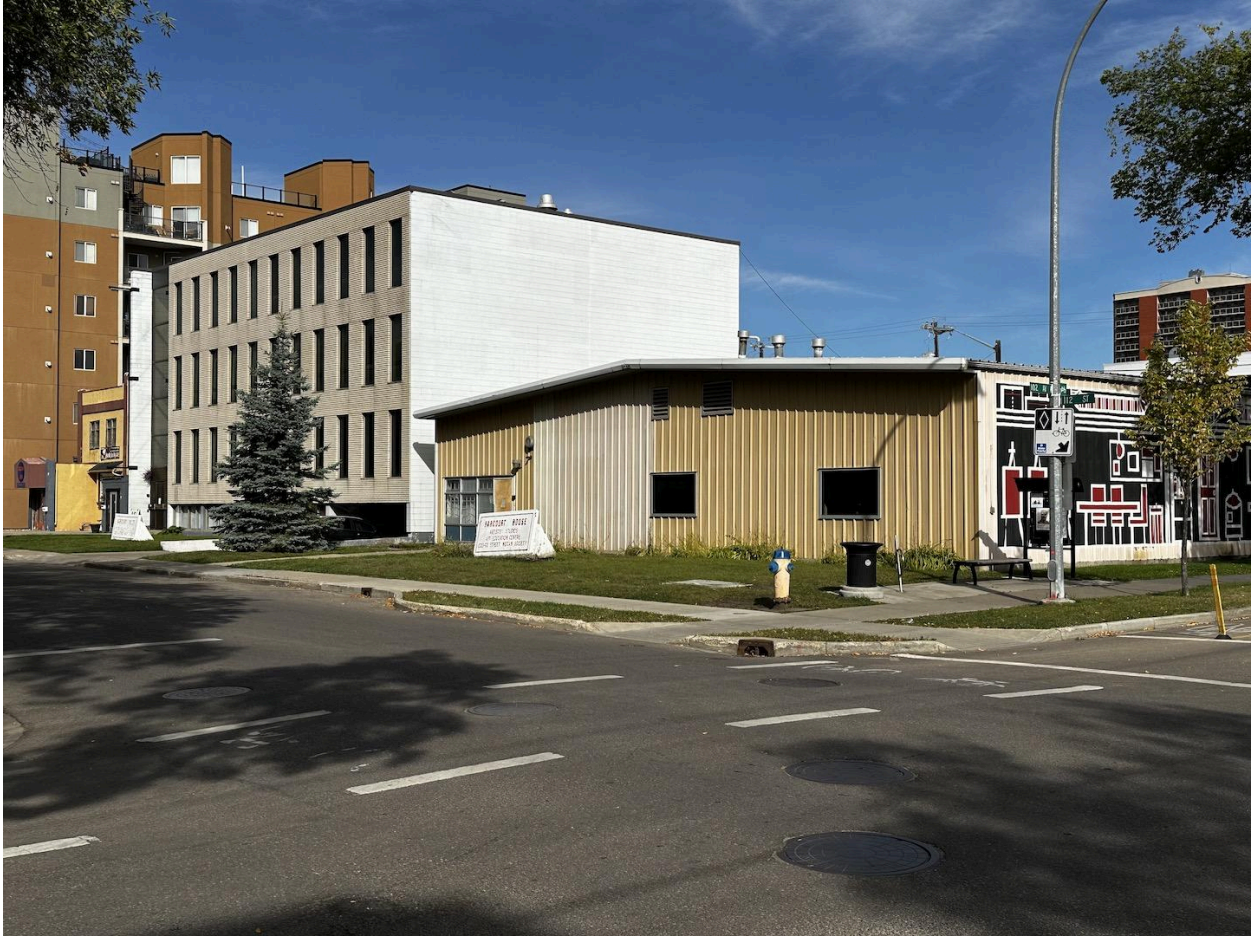
Front (west) and side (south) elevations of Harcourt House, with annex building in the foreground. The annex building is not part of the historic designation.
