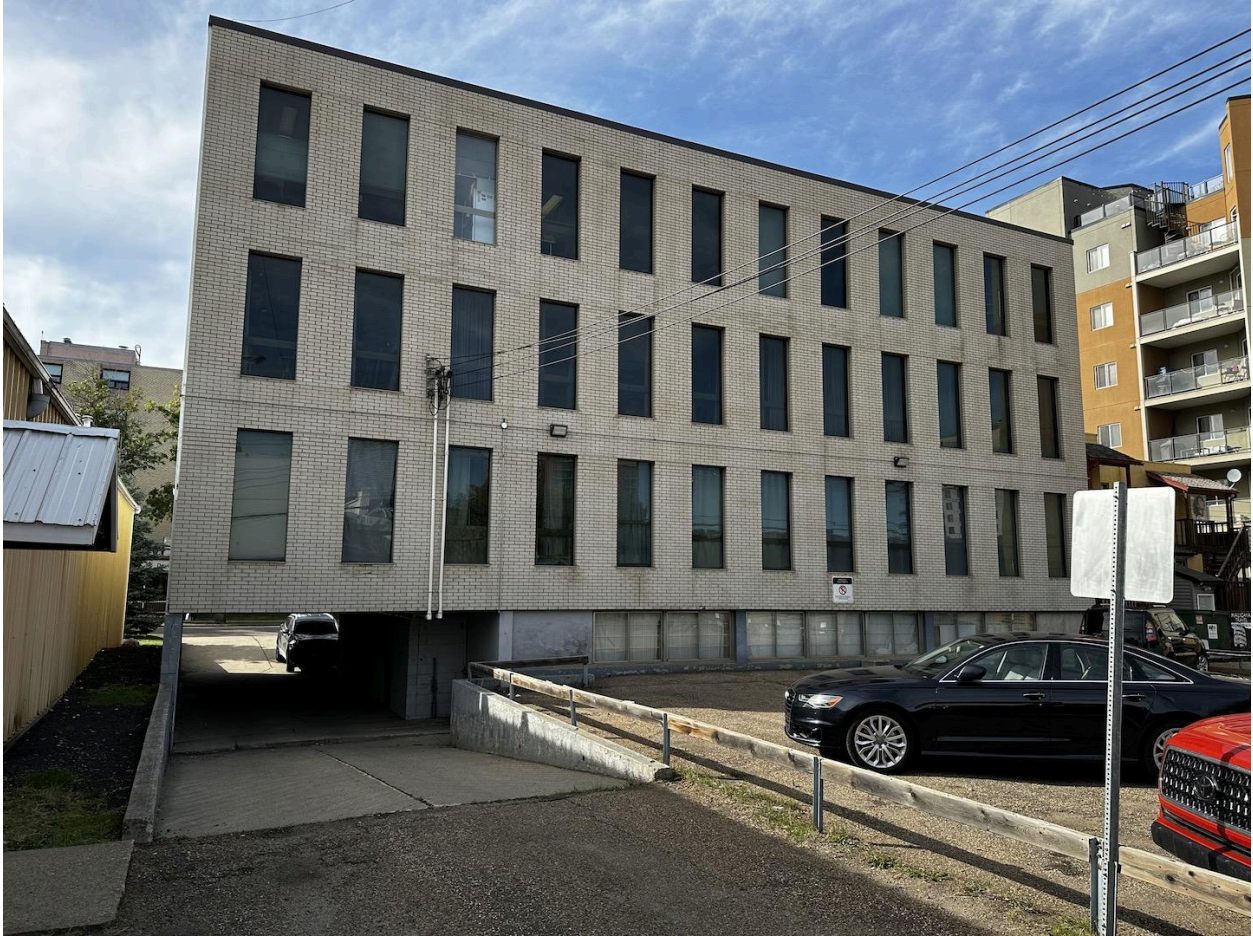
Rear (east) elevation of Harcourt House, with south driveway visible.
