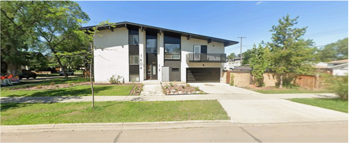
View of site looking west from 108 Street NW
