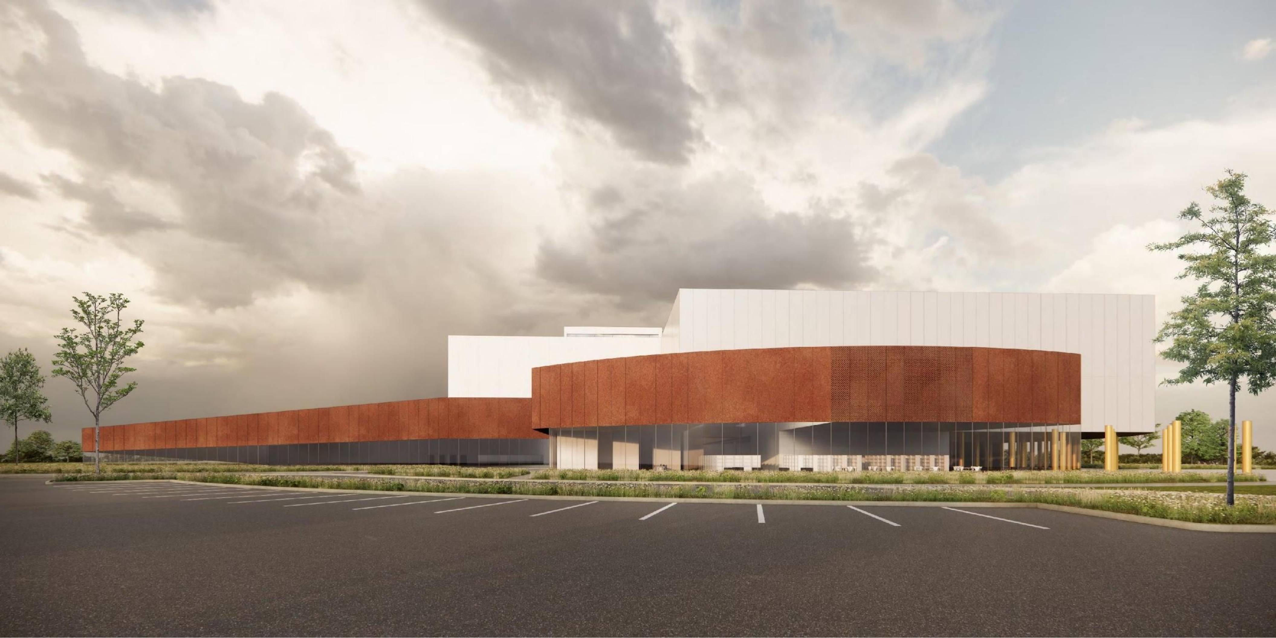
View from east looking toward the west. On the left is the Aquatic Centre, in the background is the Hub, and in the foreground is the Edmonton Public Library.
