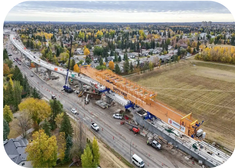
LRT - Gantry crane building the elevated guideway (87 Ave)
