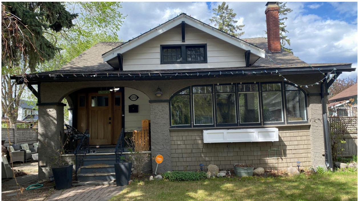
View of front (south) elevation, looking north from the front yard of the property.
