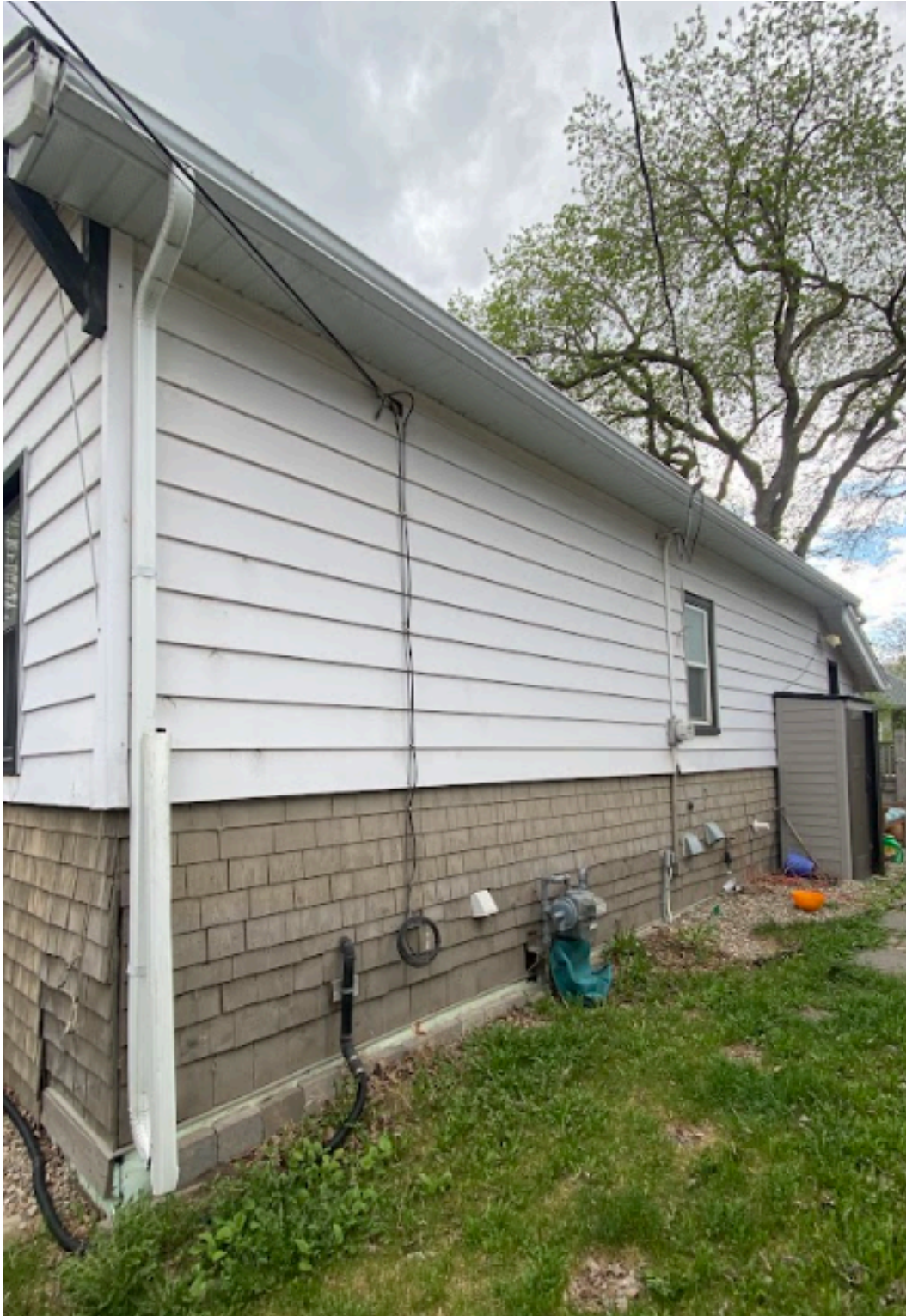
View of rear (north) elevation.
