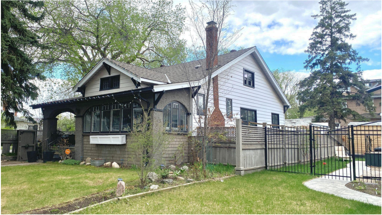
View of side (east) elevation, looking northwest.
