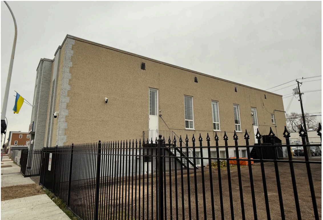
View of south elevation, looking north from 98 Street NW.
