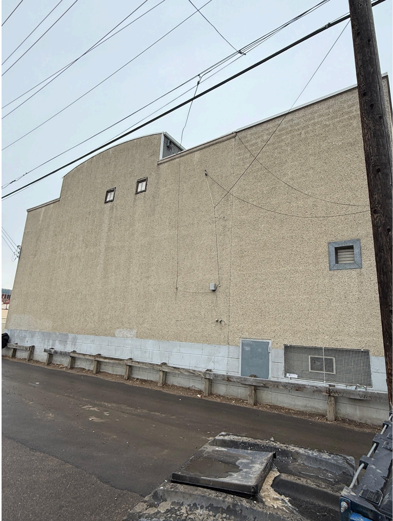
View of rear (east) elevation, looking west from rear alley.
