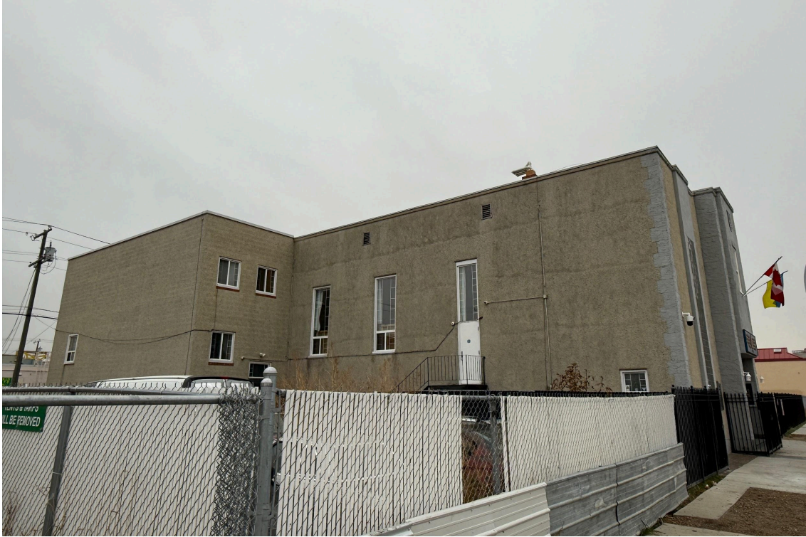
View of north elevation, looking south from 98 Street NW.
