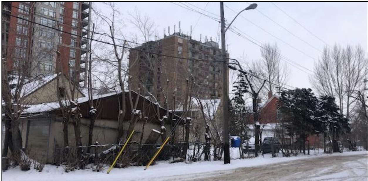
VIEW OF THE SITE LOOKING SOUTHEAST FROM THE REAR LANE
