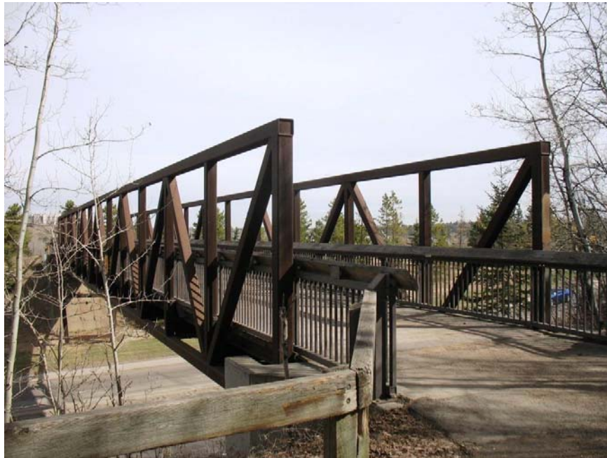
Plate 5.28. Connors Road pedestrian bridge
