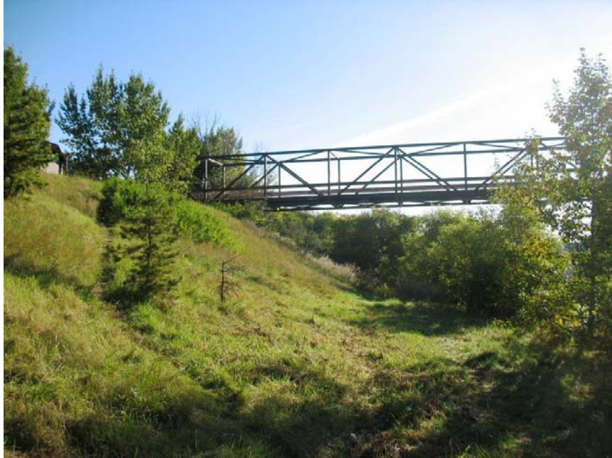
Plate 5.1. Steep slopes above the north river bank
