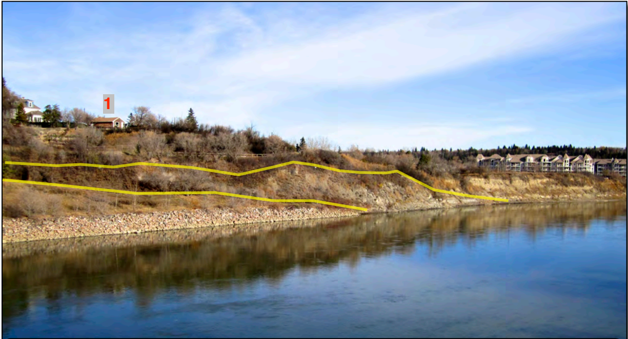
Figure 13. View facing northeast from footbridge of exposed bedrock face (bounded within — lines) along northside cutbank of North Saskatchewan River. 1 = reference point (see house in Fig. 12) proposed LRT alignment .
