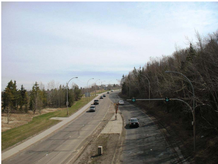
Plate 5.40. View to the east from the Connors Road pedestrian bridge
