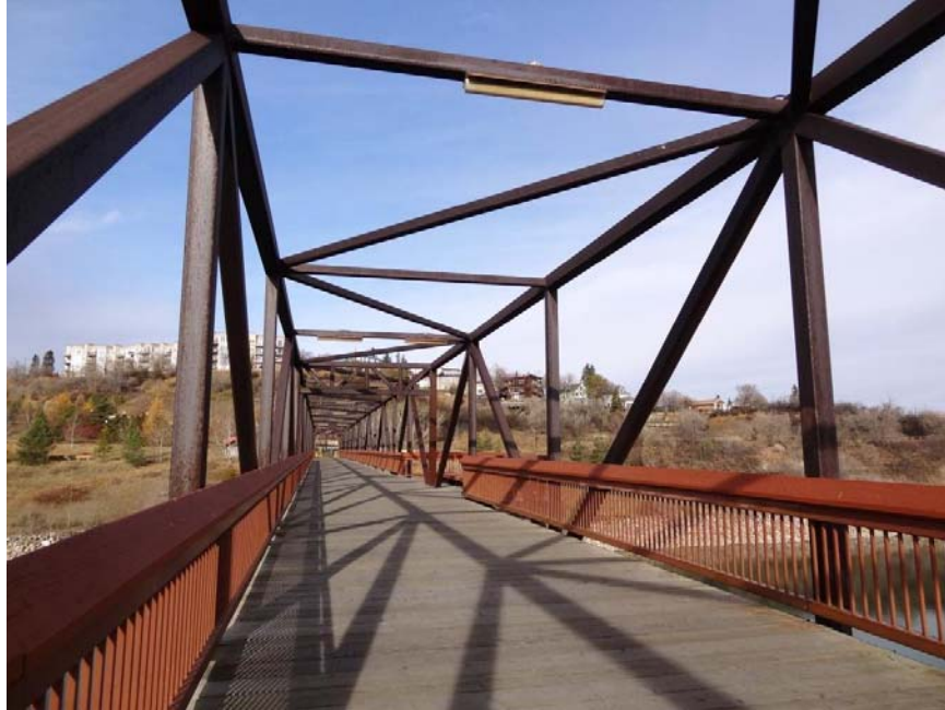
Plate 5.20. Cloverdale pedestrian bridge
