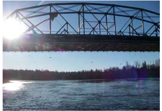
Plate 8- Looking upstream from downstream end of study section (approximately 2 km downstream of Cloverdale Bridge).
