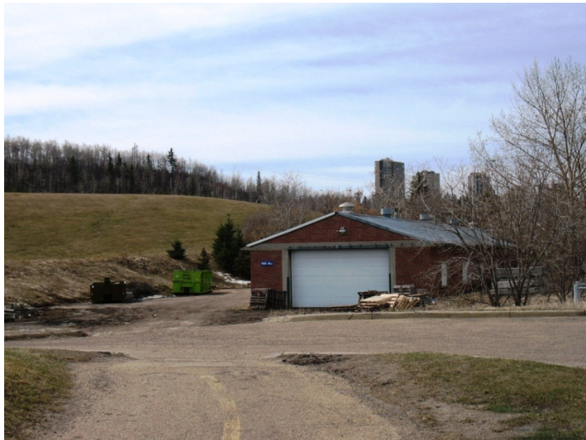
Plate 5.25. Muttart storage facility
