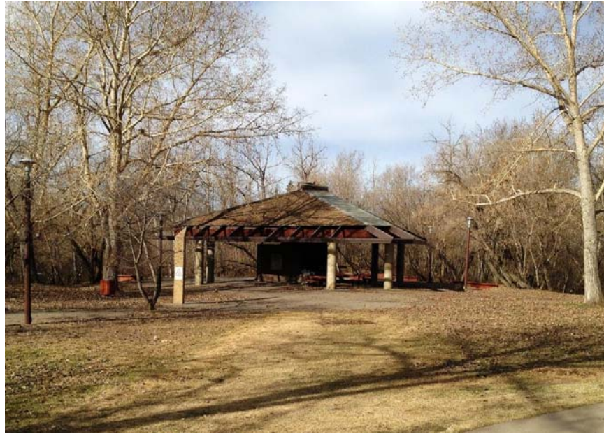
Plate 5.21. Picnic shelter at HME Park
