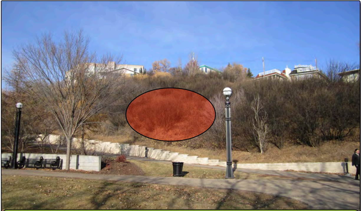
Figure 11. View facing north from pedestrian walkway on north bank of North Saskatchewan River Valley showing approximate LRT tunnel portal (●) placement.
