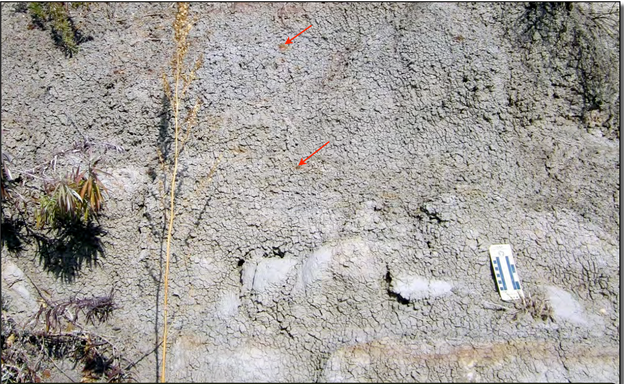
Figure 15. Close-up of weathered bedrock face in Fig. 14 showing interbedded layers of siltstone/mudstone, silty sandstone and ironstone fragments (→) in slopewash .
