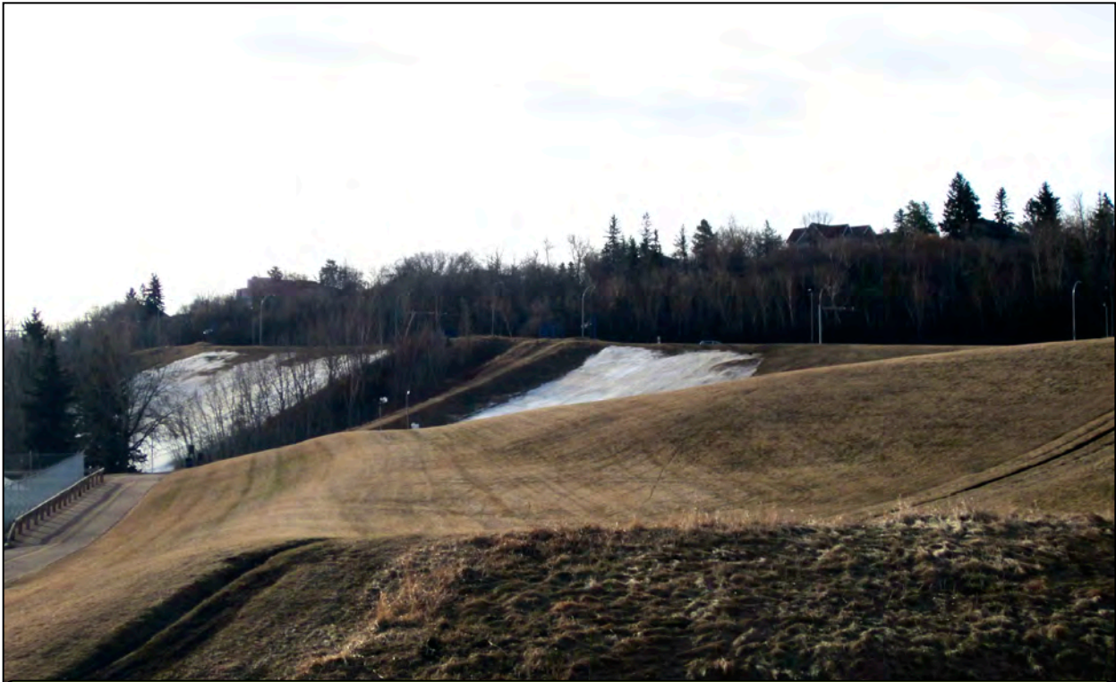
Figure 28. View looking southeast below Connors Road showing moderate to steep landscaped slopes along the middle valley slope. Area of thin cover over bedrock.
