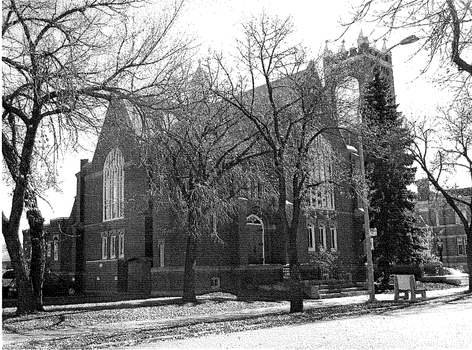
View of north and west elevations
