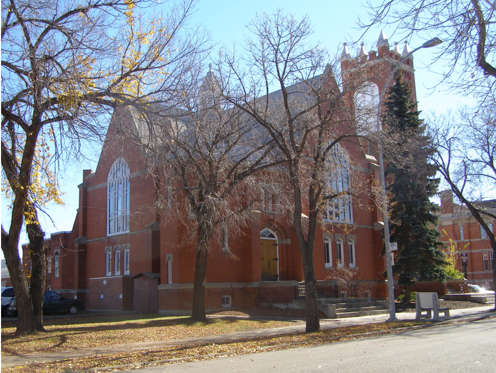
View of north and west elevations
