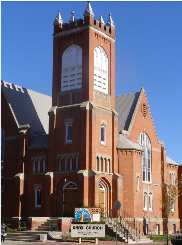
View of front entrance
