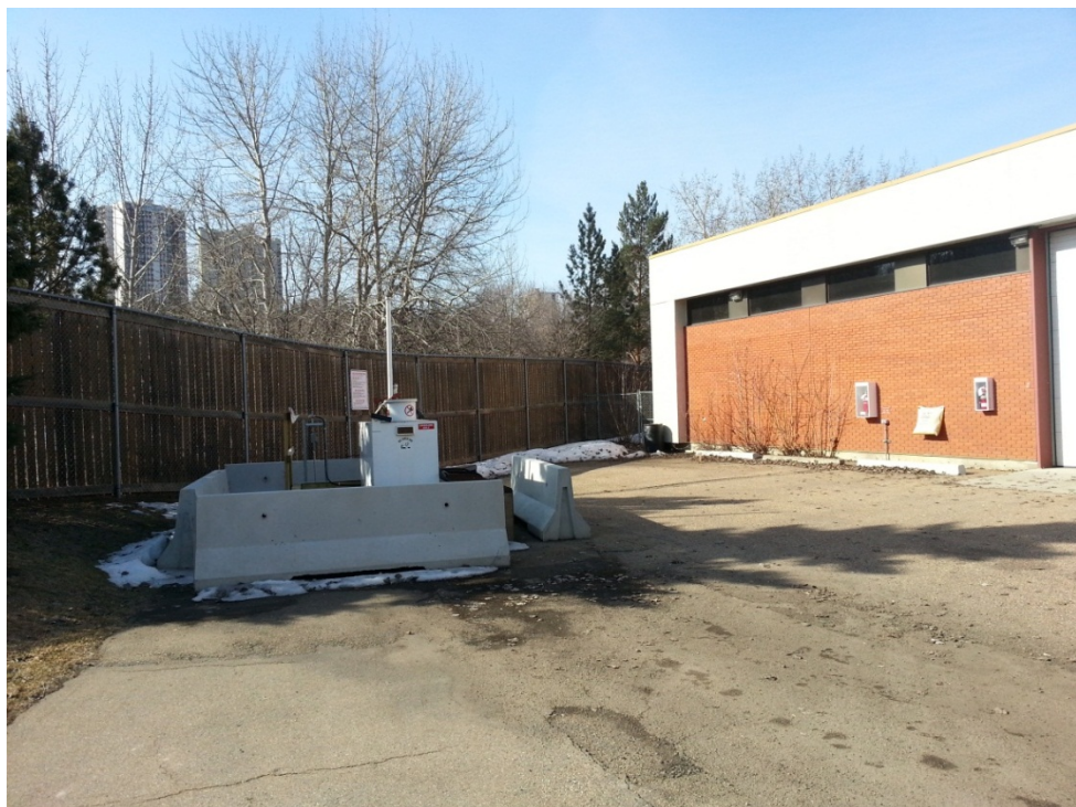
Photo 6: South-east corner of Station 21 at the location of the fueling station
