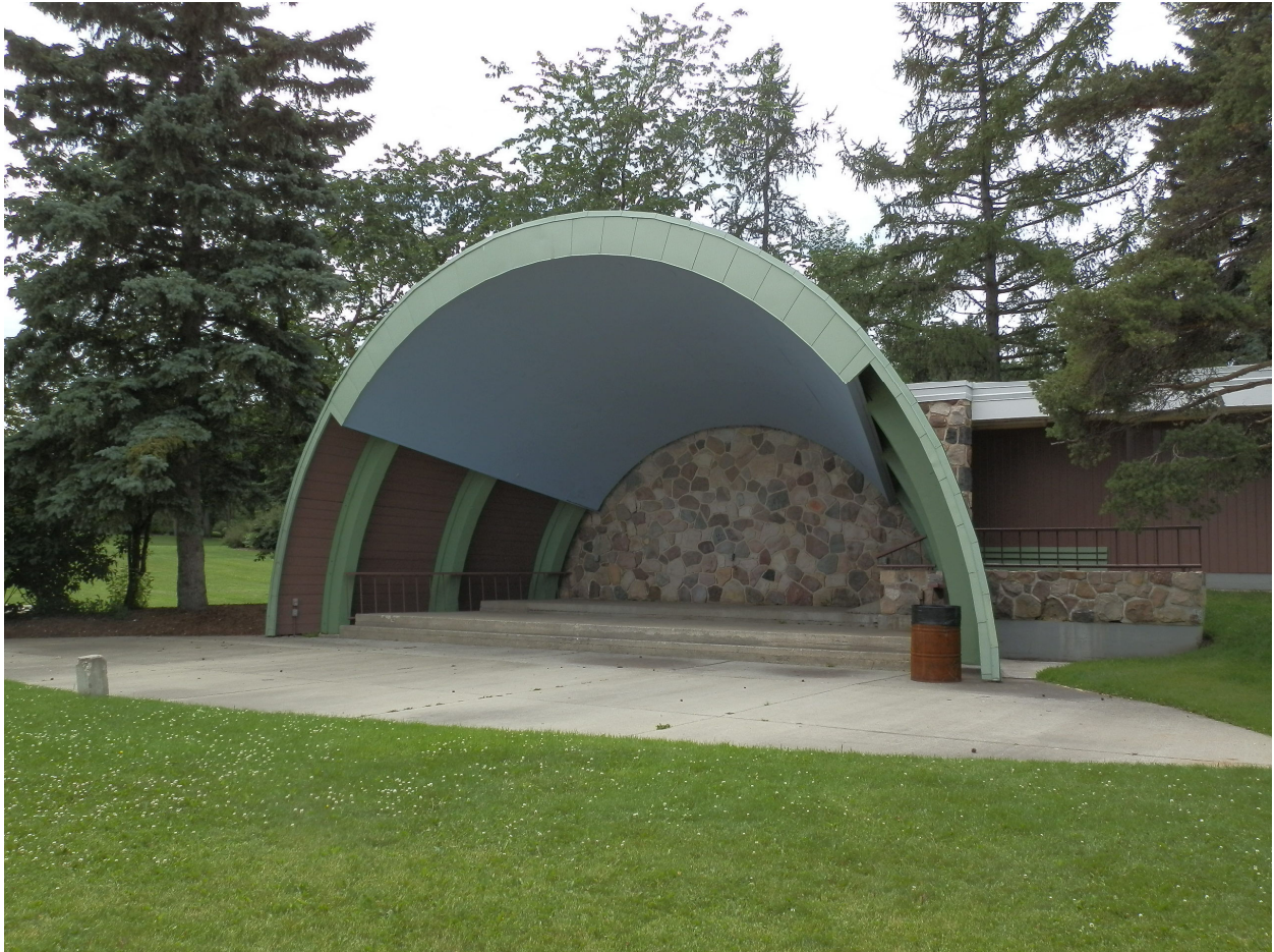
Front view of Borden Park Band Shell with wood ancillary building in background
