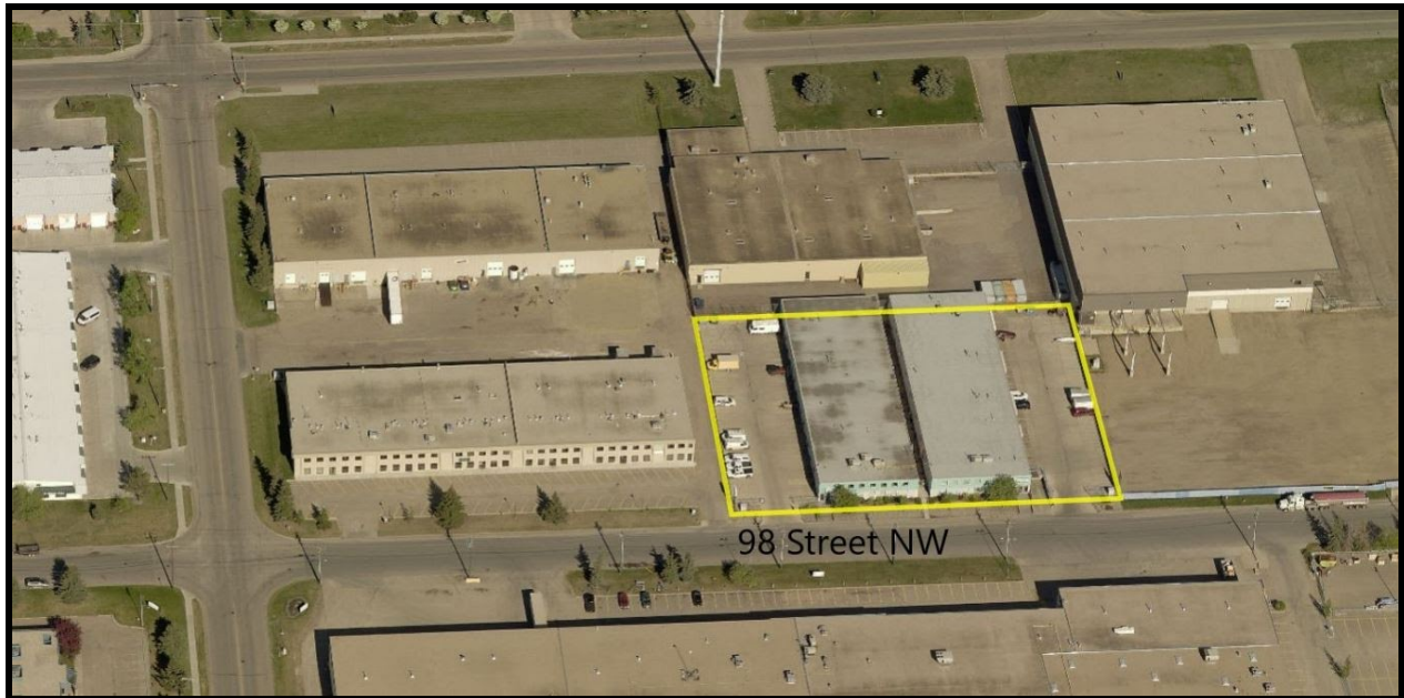
VIEW OF SITES LOOKING EAST
