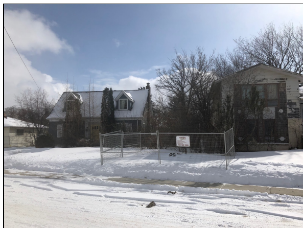
VIEW OF SITE LOOKING SOUTH
