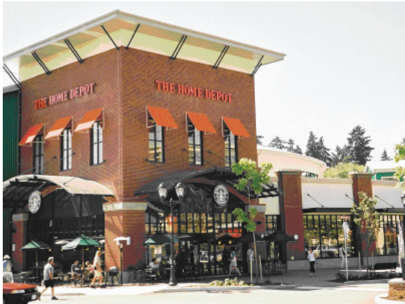
Figure 86: Station Hub Retail–Hardware Store
