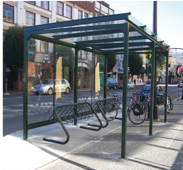
Figure 63: Covered Bicycle Parking
