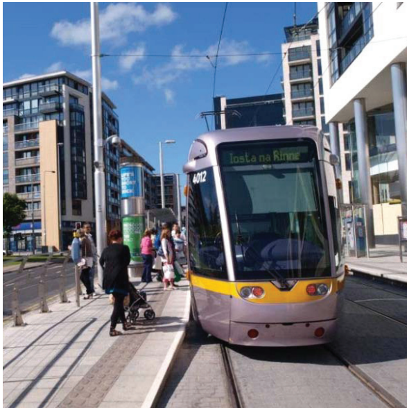
Figure 24: Low-Floor LRT Station - Dublin, Ireland
