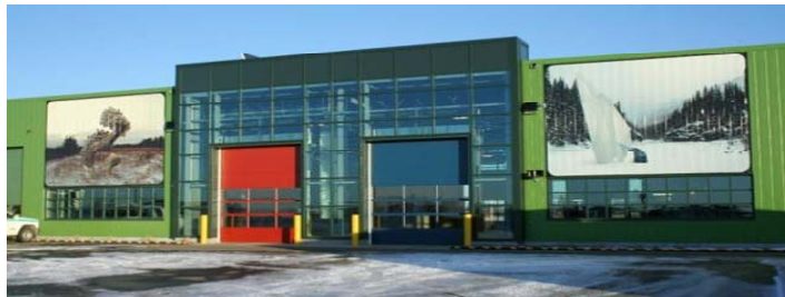
Ambleside Eco Station shown here is the template for NE Eco Station
