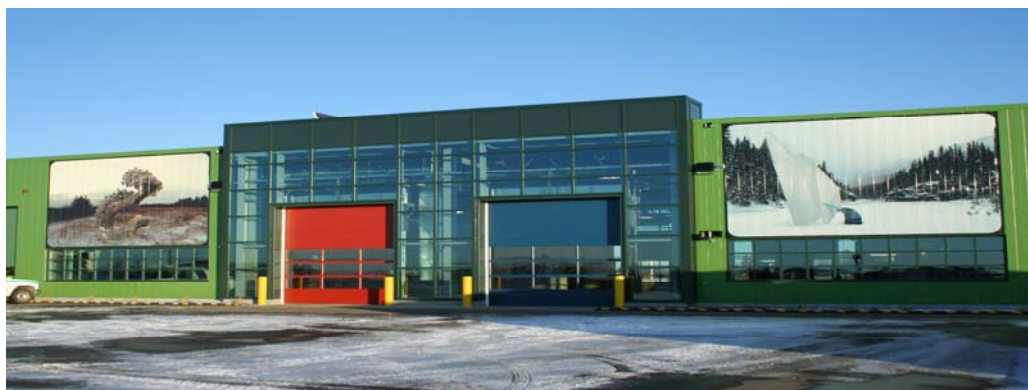
Ambleside Eco Station (Template for Northeast Eco Station)
