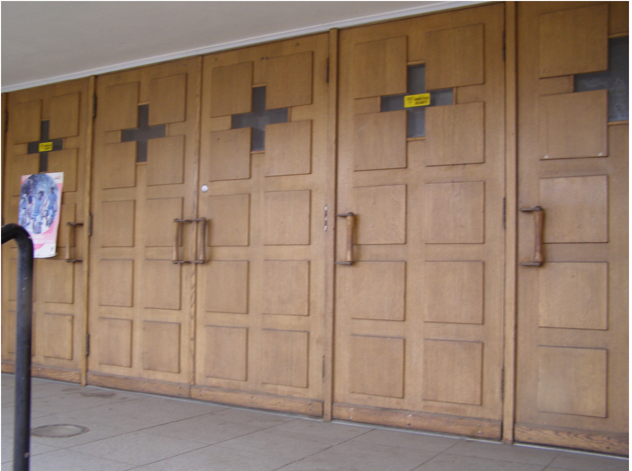
Detail of front entrance doors
