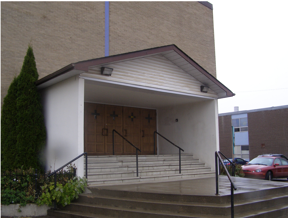
Front entrance of church
