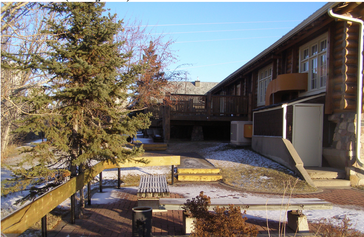
West elevation (looking north)
