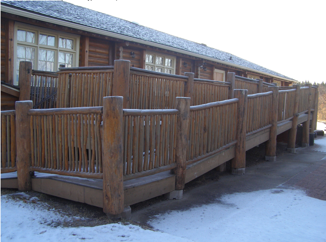
West elevation (looking south)
