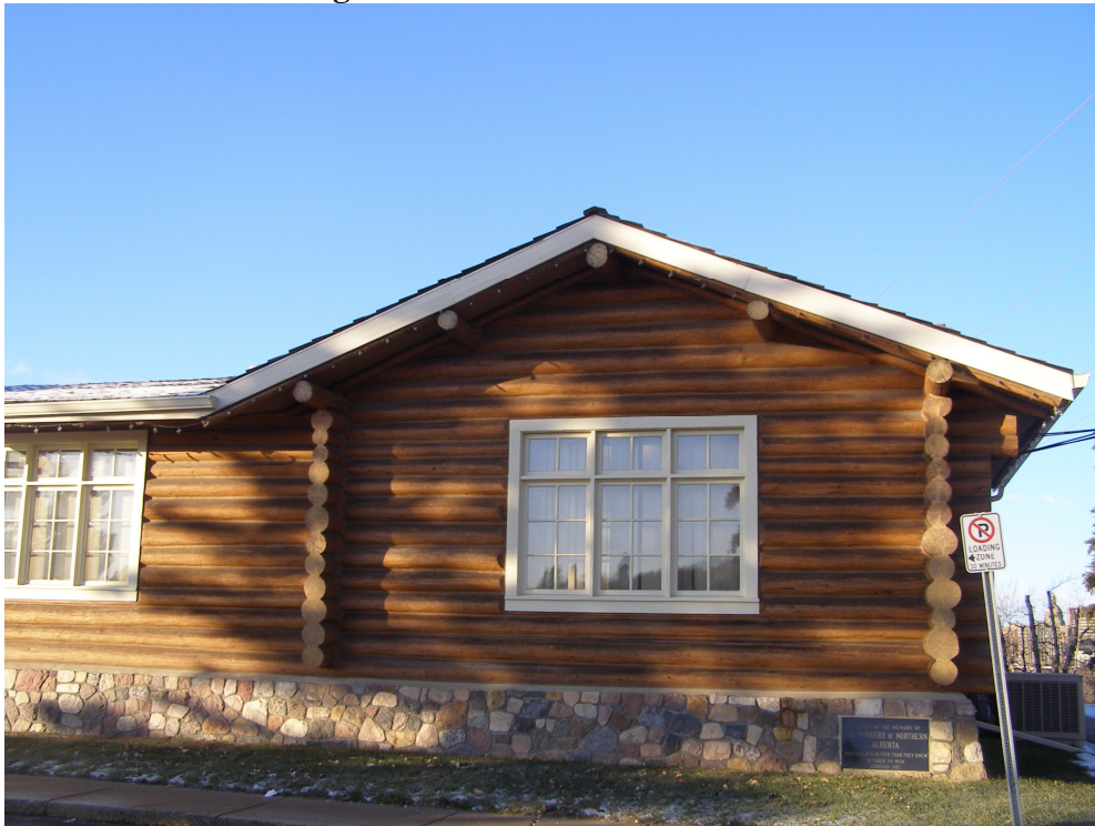
East elevation showing the 1987-88 addition
