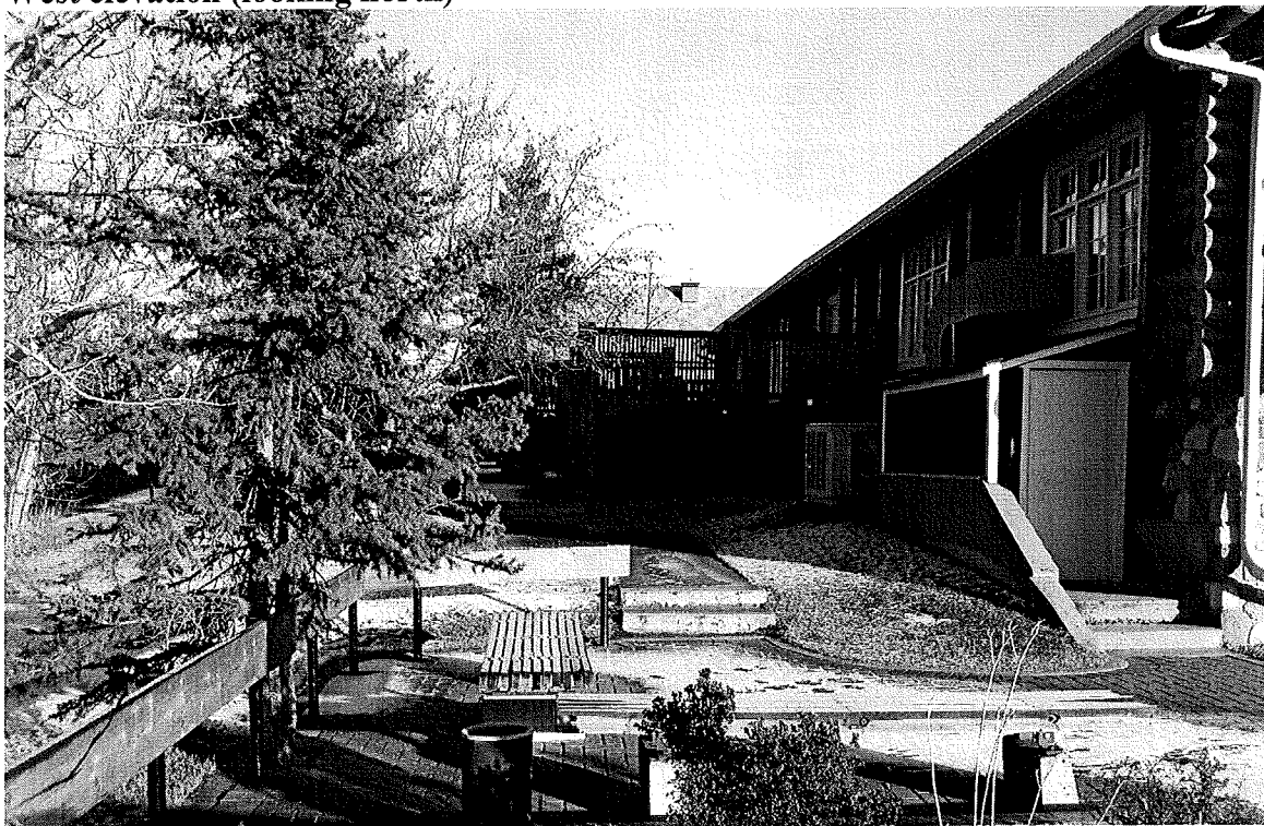
West elevation (looking north)
