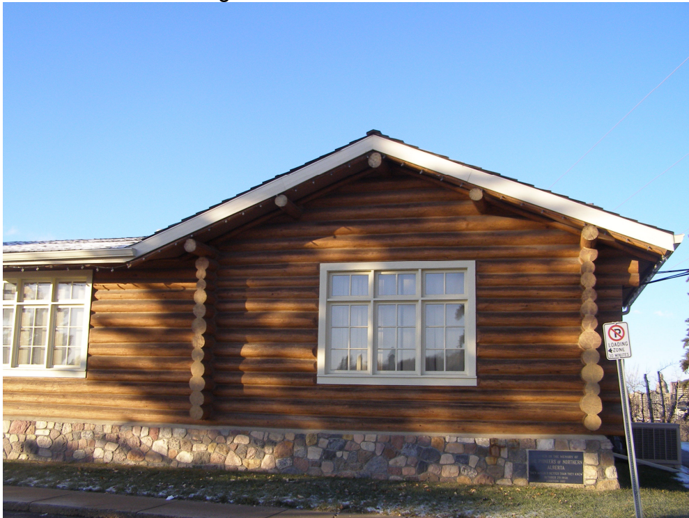
East elevation showing the 1987 - 88 addition
